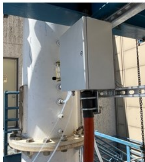
New Membrane Drier and Heated Sample Line for Outlet \text{SO}_2 Measurements
