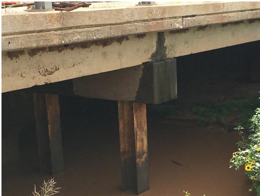
Figure B. 2: Corroded bents under China Creek bridge to be replaced
