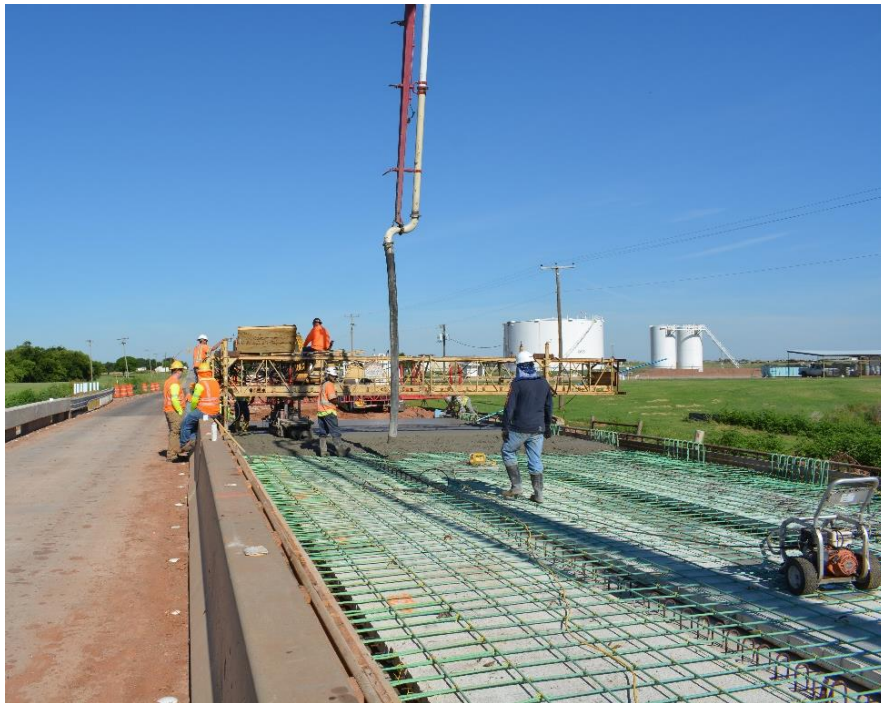
Figure B. 44: Phase 2 deck concrete placement
