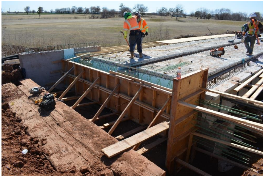
Figure B. 11: Forming of abutment walls after placement of girders and precast panels, March 2020 (East abutment)
