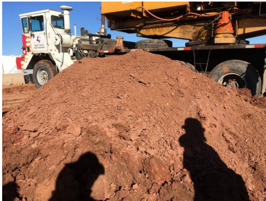
Figure B. 9: Heap of soil excavated from the drilled shaft. Note the broken pieces of shale on top (depths of 7.5 m and lower) and wetter/plastic material removed beforehand
