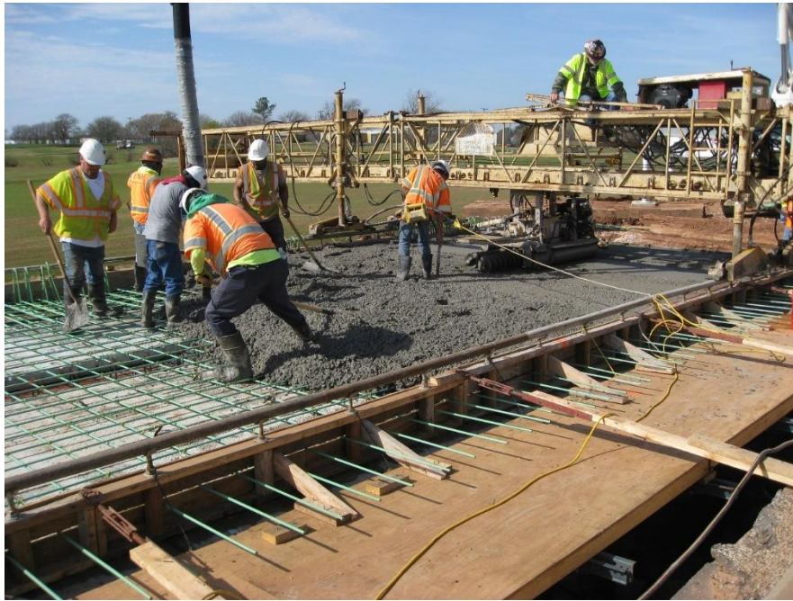
Figure B. 19: Concrete placement on the deck, Phase 1, March 2020
