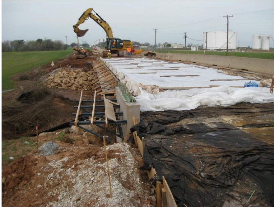
Figure B. 21: Covered deck surface after concrete was placed, Phase 1, March 2020
