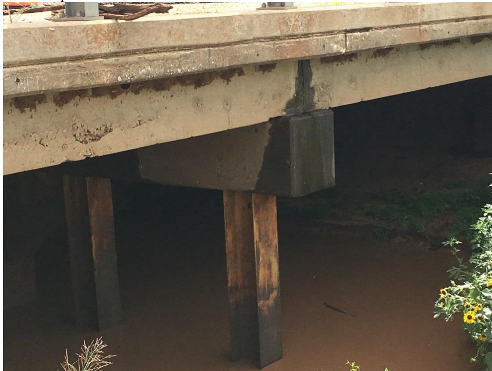
Figure 1. 2: Seepage of surface runoff through the bridge expansion joint between two adjacent spans in China Creek Bridge, Wichita County, TX
