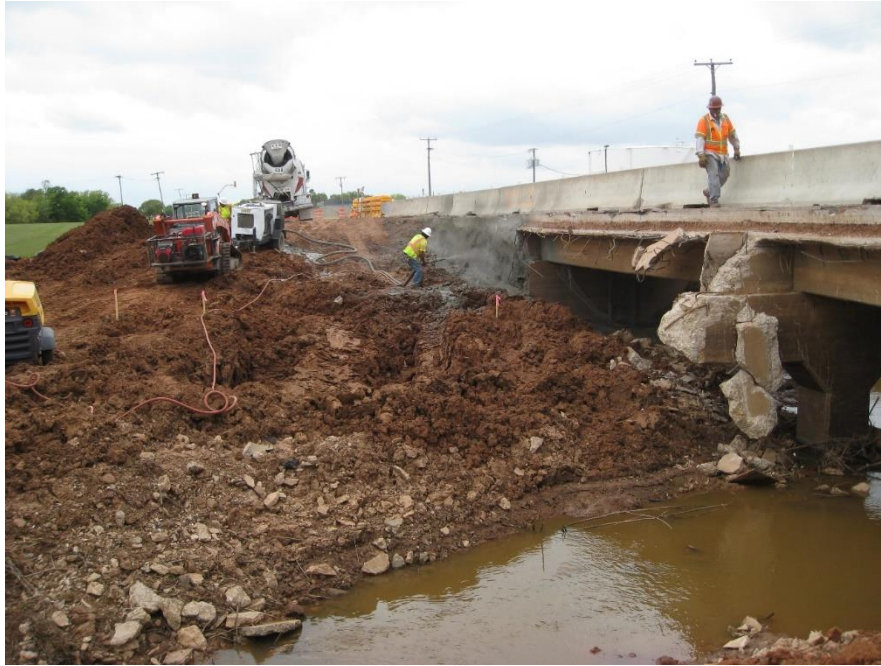
Figure B. 6: Installation of soil nail wall as temporary support for the active roadway crossing the undemolished half of the bridge (Picture provided by Samuel Groves)
