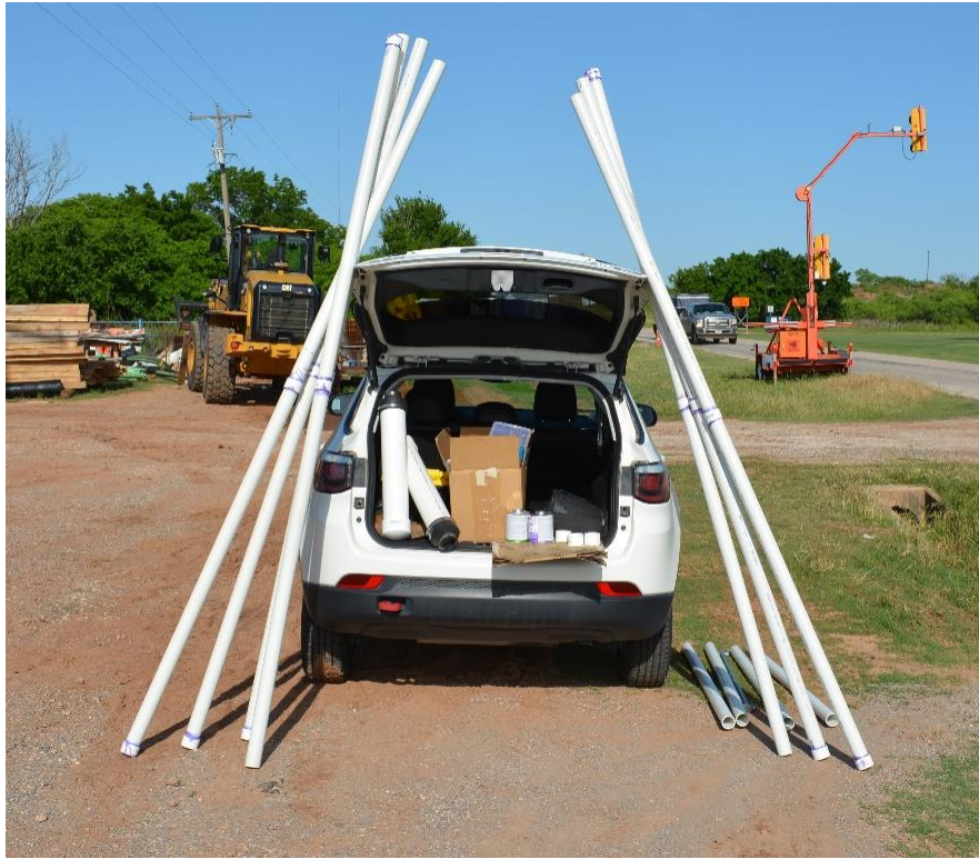
Figure B. 22: 1.5 m PVC conduits transported to China Creek Bridge to house SAAV sensors in the drilled shafts. In this picture, 1.5 m conduits are already assembled into 3 m sections using PVC cement and couplers
