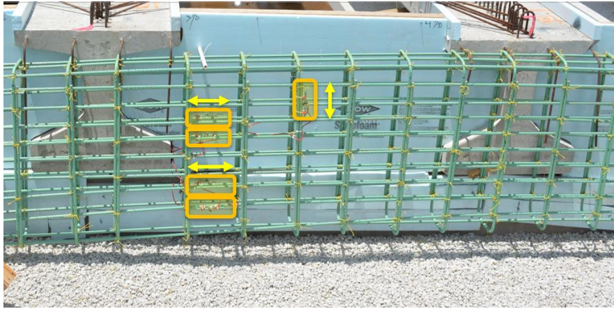
Figure B. 41: Location of the 3 pairs of concrete embedded strain gauges on the east abutment wall
