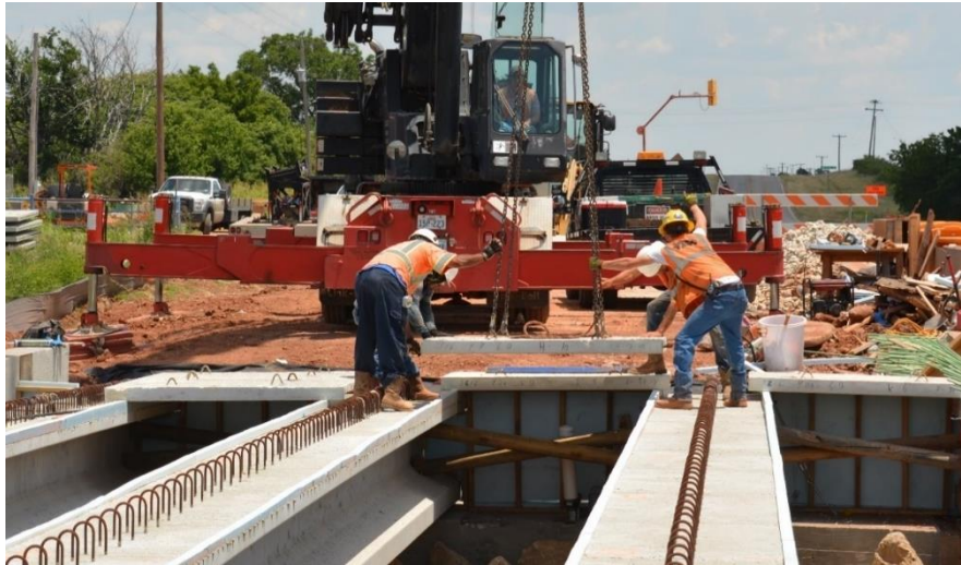
Figure B. 43: Placement of precast concrete panels on the deck
