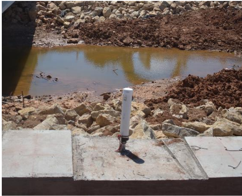
Figure B. 37: Capped SAAV conduit on east abutment
