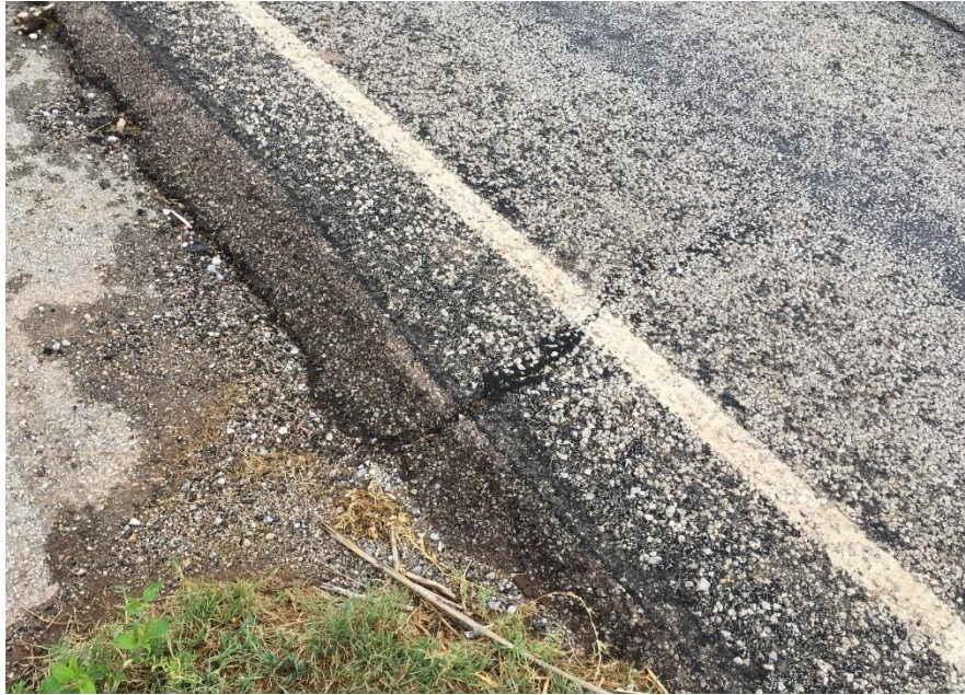
Figure B. 4: Cracked edge of pavement at the end of the approach slab due to backfill settlement
