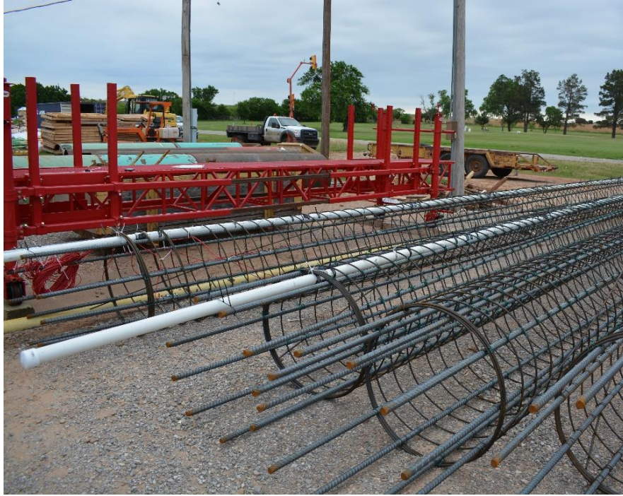
Figure B. 26: Assembled PVC conduits attached to drilled shafts to serve as SAAV housing
