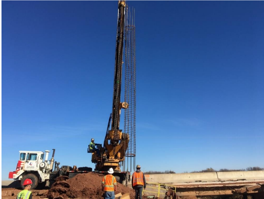
Figure B. 10: Placement of one of the west abutment drilled shafts' rebar cage
