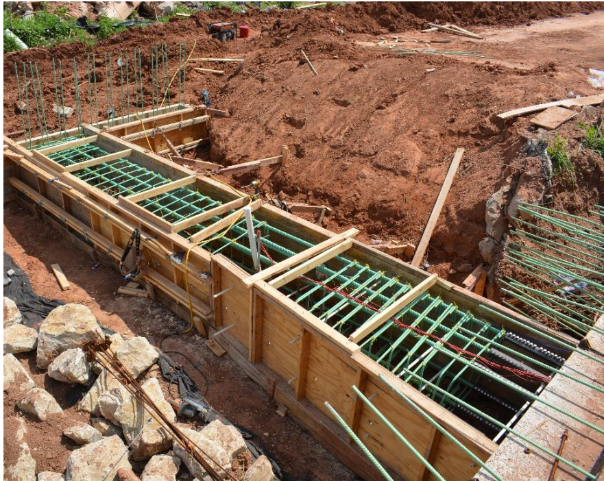
Figure B. 31: Formwork for construction of abutment caps and wing walls
