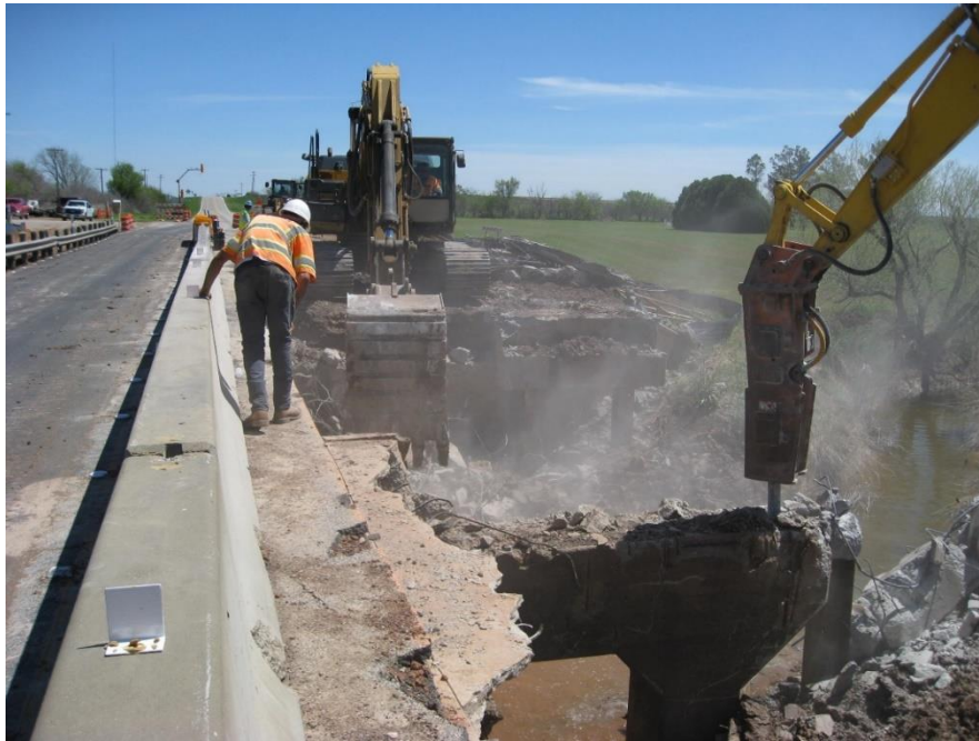
Figure B. 5: Demolition of the first half of the old China Creek Bridge
