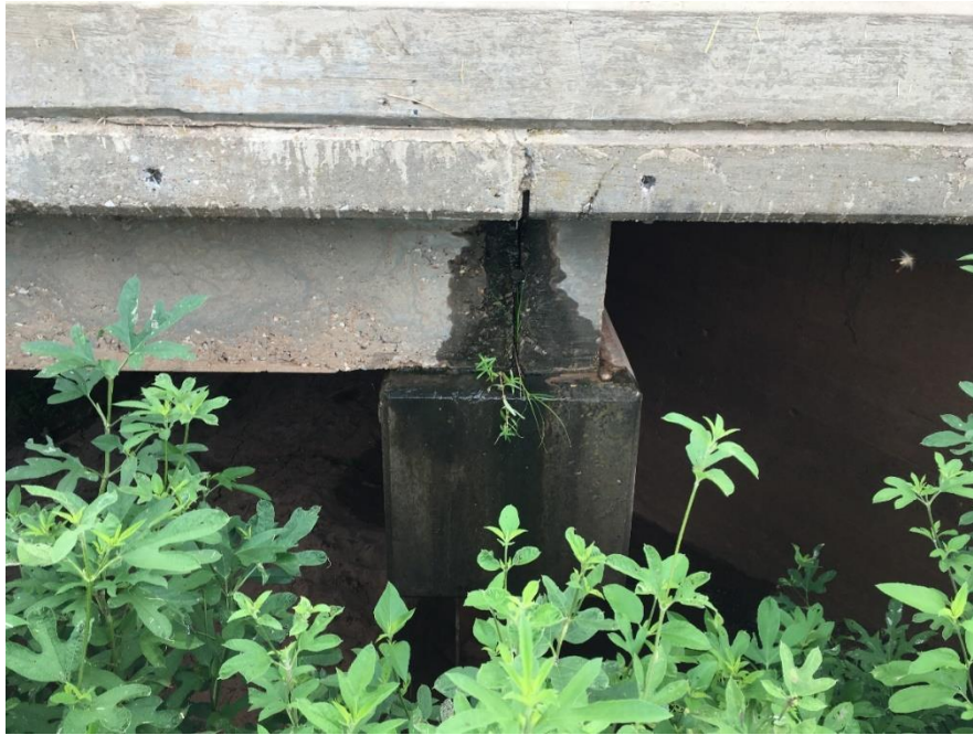
Figure B. 3: Seepage of water through the deck joints
