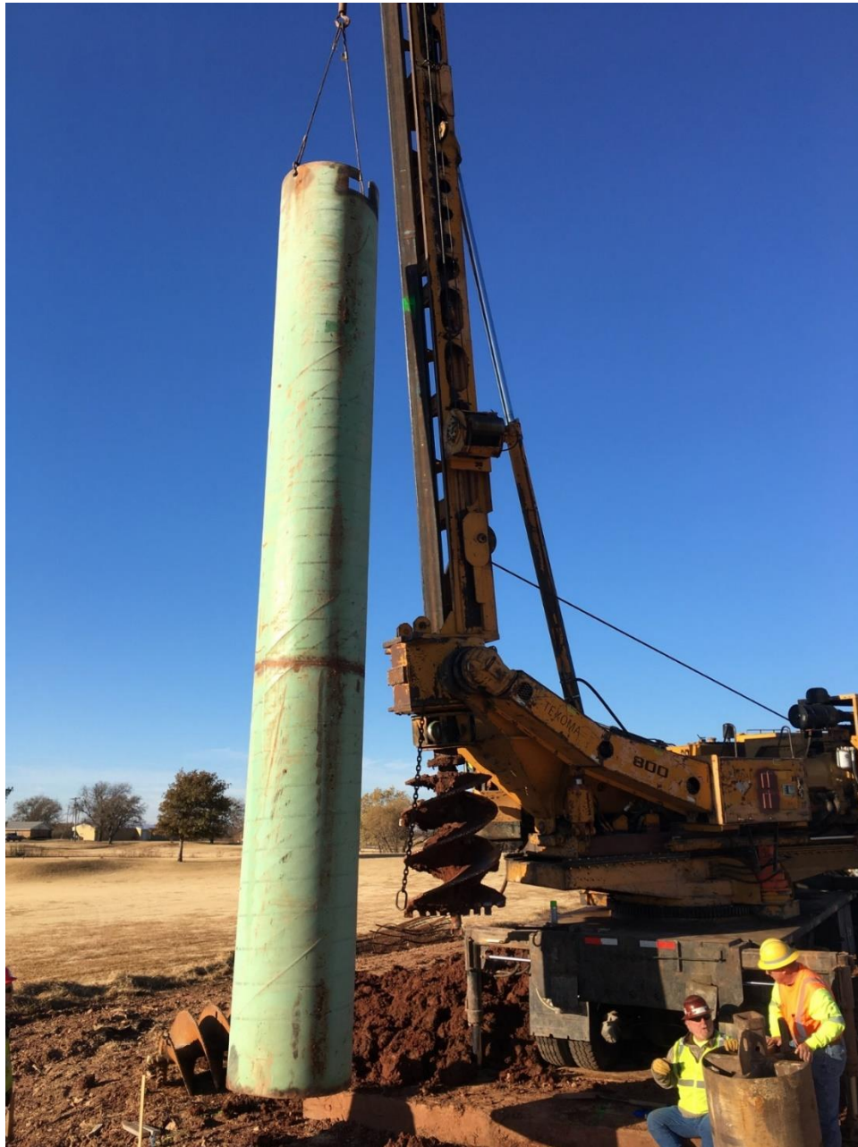
Figure B. 7: Casing used for the top portion of the drilled shafts
