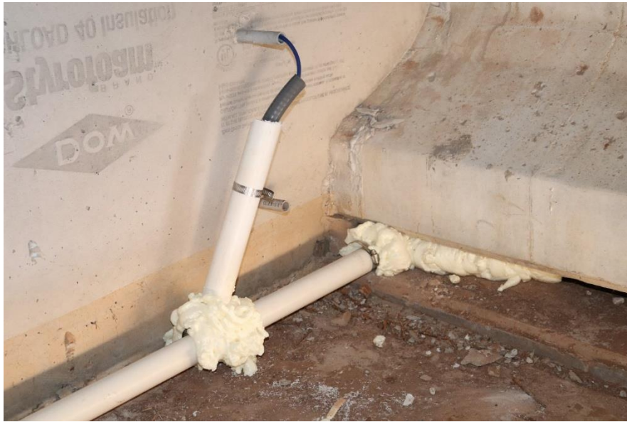
Figure B. 60: PVC pipes used for protection of cables routed on top of abutment caps
