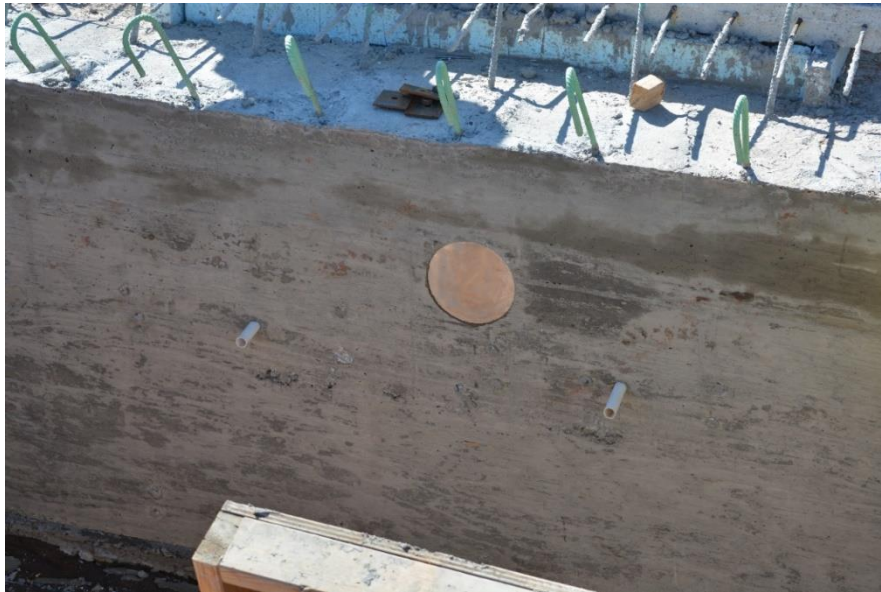
Figure B. 13: Finished surface of the east abutment wall with the pressure cell (GK-4810) installed between the two girders on the left, March 2020
