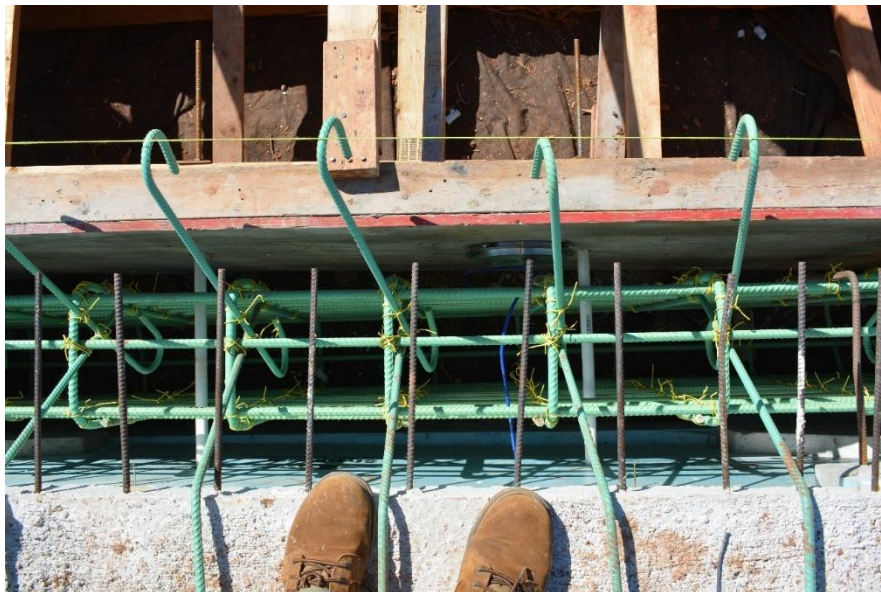
Figure B. 12: Top view of the earth pressure cell (GK-4810) installed on the inside of the form on the west abutment wall, photographer standing on one of the precast panels placed on the deck, March 2020
