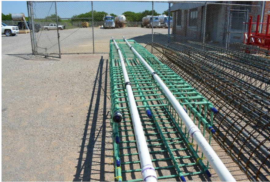
Figure B. 23: PVC conduits assembled into 11 m sections using additional couplers and joint reinforcement.
