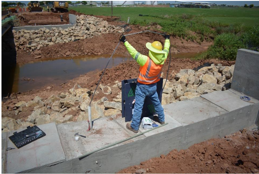
Figure B. 35: Installation of SAAV in the east abutment center drilled shaft
