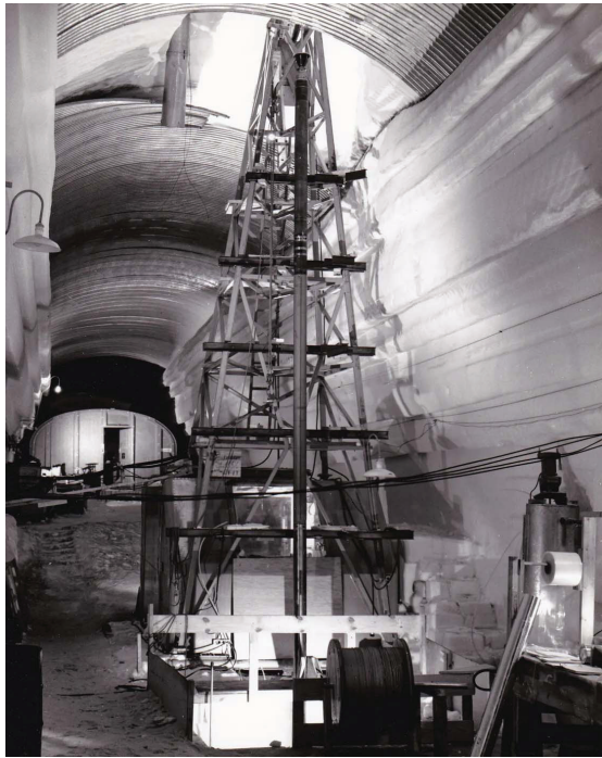
Figure 22 Century site drilling equipment.
