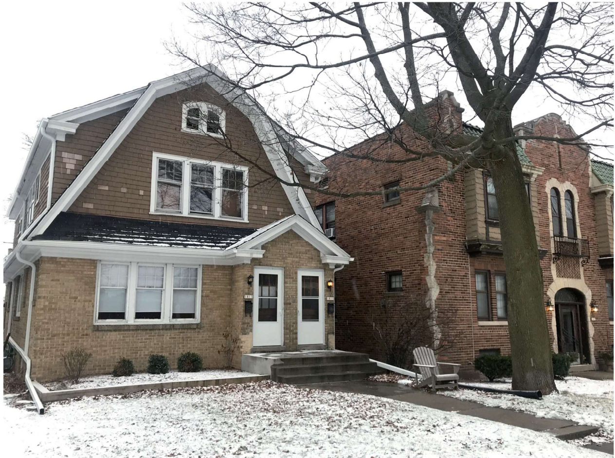
Figure 1. A side-by-side duplex (left) and small apartment building (right) in Shorewood (WI) are examples of “Missing Middle” housing. Source: Sightline Institute Missing Middle Homes Photo Bank.
