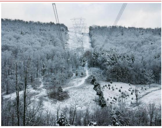
It was the first leg in what today is a network of 765-kV lines extending for more than 2,000 miles. The highest-voltage line in operation until that point was a 735,000-volt line in Canada. One 765,000-volt line can carry as much power as five 345,000-volt lines or as many as thirty 138,000-volt lines.
