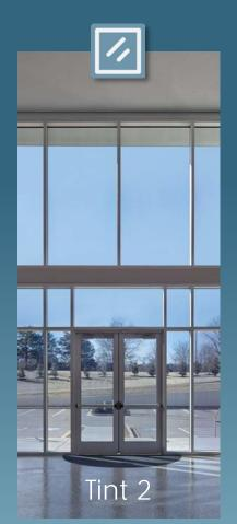
Visual light transmission: 30% Solar heat gain coefficient: 0.23
