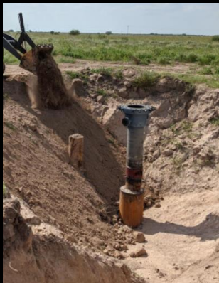
Re-enter gas exploration well
