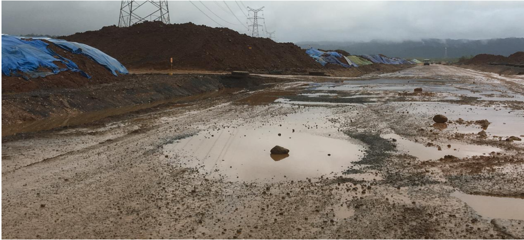
Figure 5: Tailing deposit on the road, Konawe (author's field research 2019)
