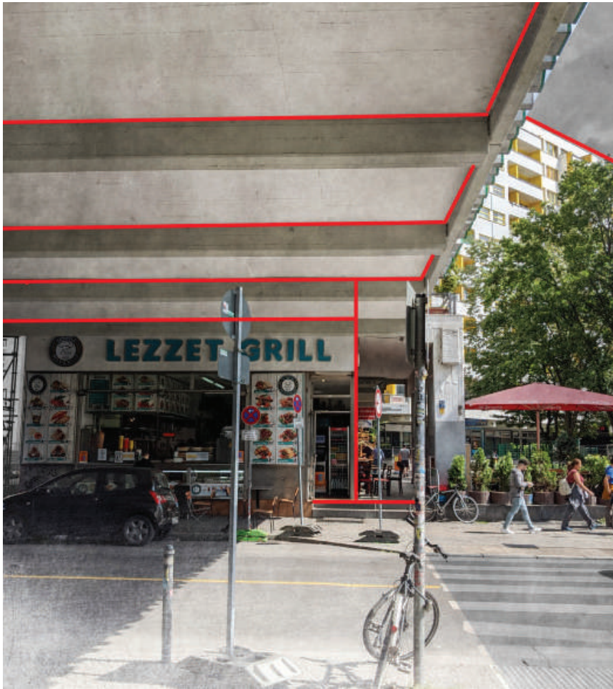
03 Turkish Food Restaurant under NKZ at point a to b.
