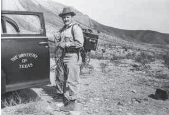
Peter T. Flawn carrying an old LaCoste & Romberg gravity meter during a gravity survey of the Hazel Mine area in Culberson County, Texas, 1951 (Photo courtesy Tyrrell Flawn)
