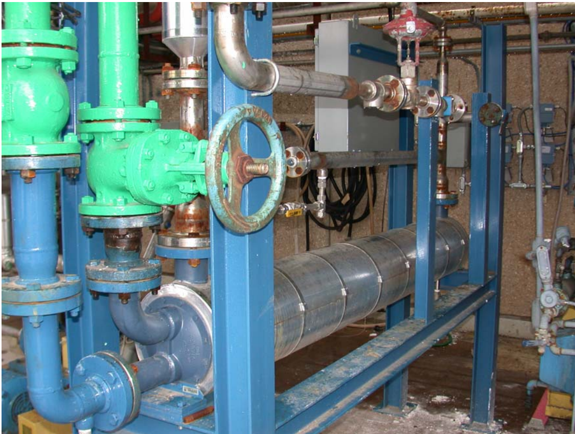
Figure 2-7. Solvent Cooler (H-107) Installed on Support Rack. Cooling Water Piping (Green) Flows Tube Side (Picture Taken by C. Lewis)
