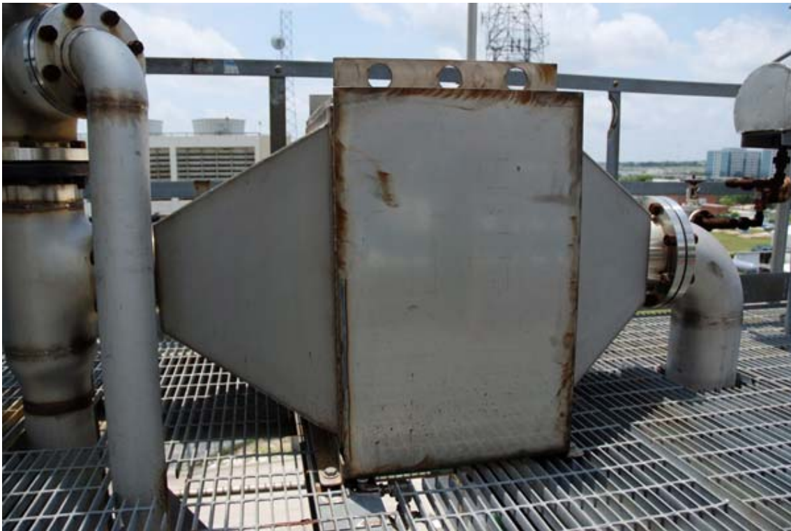
Figure 2-8. Air Cooler (H-112) Installed on Top Platform of Structure. Radiator Coils are Located on the Opposite Side (Picture Taken by C. Lewis)
