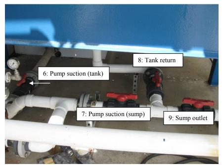
Figure A.3. Liquid line valves (south).
