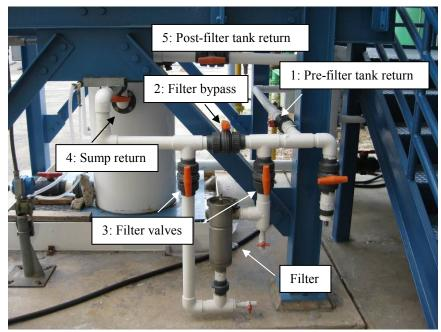
Figure A.2. Liquid line valves (north).
