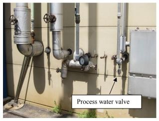
Figure A.1. Process water source.
