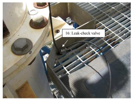
Figure A.9. Leak-check valve.
