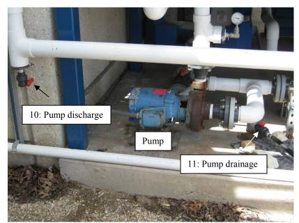
Figure A.4. Pump and associated valves.
