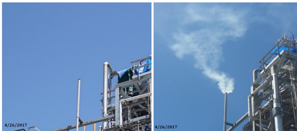
Figure 1.3: Large plumes of PZ aerosol observed after 52 ppm \text{SO}_3 injection at the April 2017 UT-SRP pilot plant campaign. Photos by Beaudry (Beaudry, 2017).
