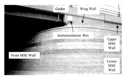
Fig. 1. View of the South-East Side of the Completed Founders/Meadows Bridge
