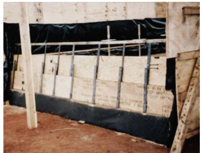
Figure 2. Photograph of wood lagging board supports used during construction
