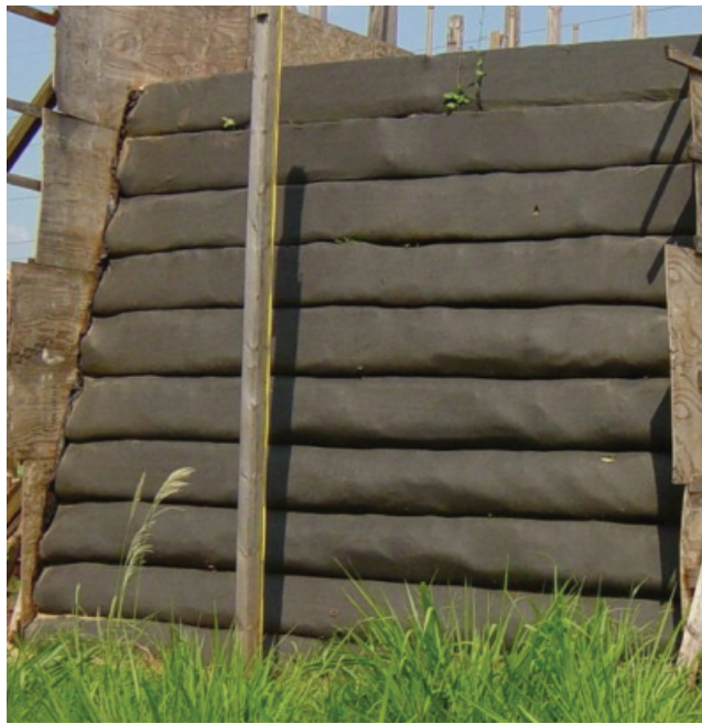
Figure 5. Front view of prototype wall 1
