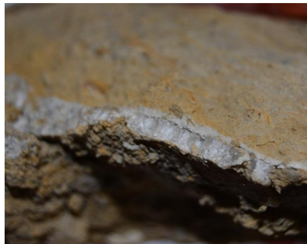
Figure 5.8.5: Gypsum seam identified in southbound locations.
