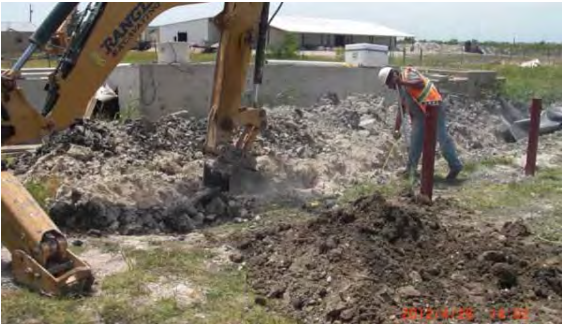
Figure 4.31: Compacting soil with backhoe bucket.
