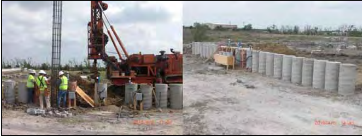
Figure 4.14: Construction of test wall, April 2010.
