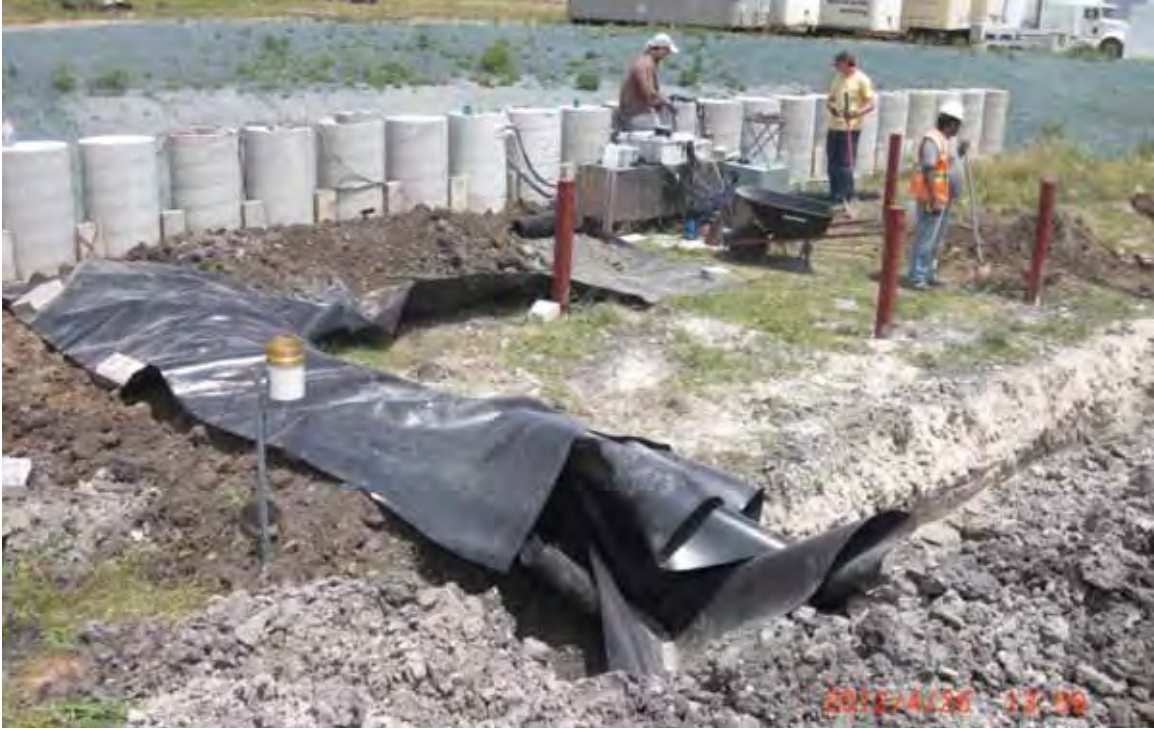
Figure 4.30: Installation of geomembrane in trench.
