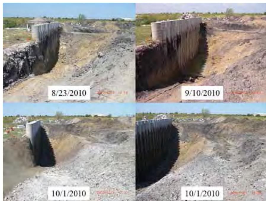
Figure 5.6: Photos of later excavation progress (8/23/2010 - 10/1/2010).
