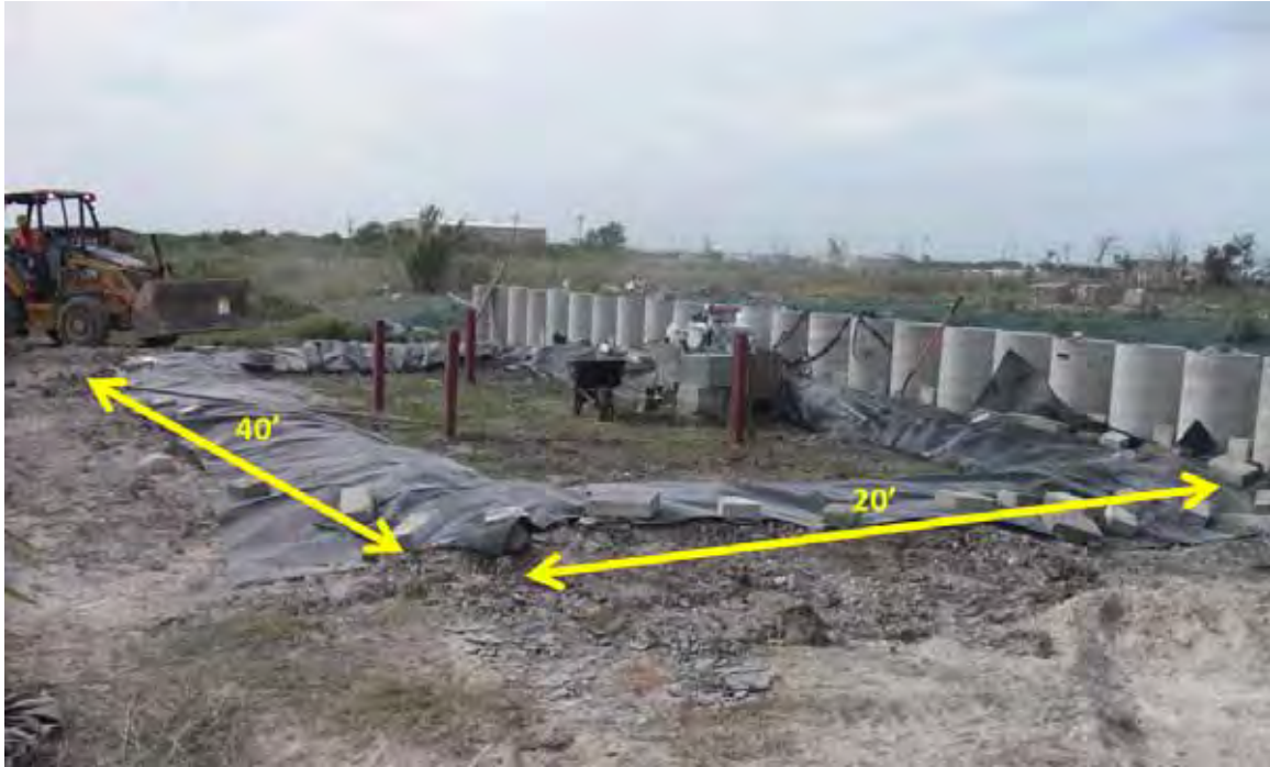
Figure 4.34: Completed inundation berm.
