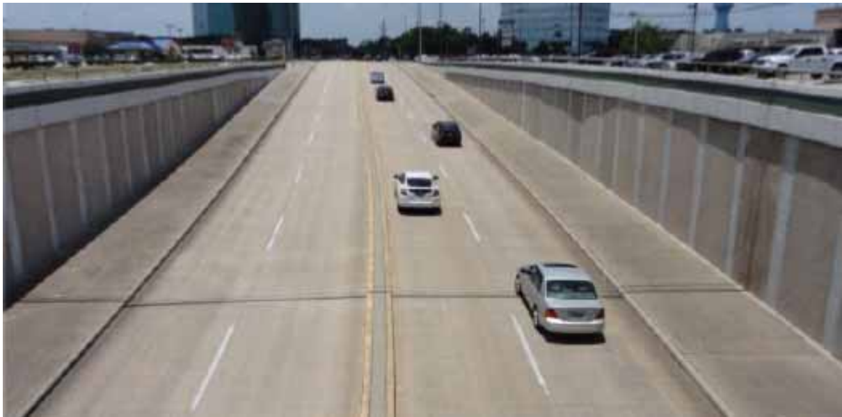
Figure 3.35: View of current wall conditions, facing west.
