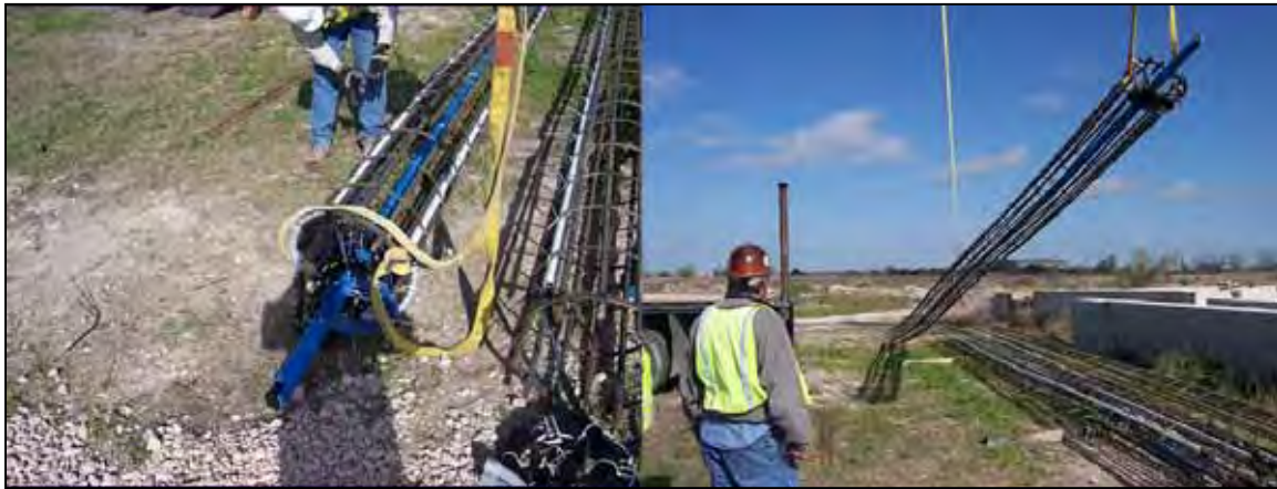
Figure 4.15: Lifting an instrumented cage with two cranes.
