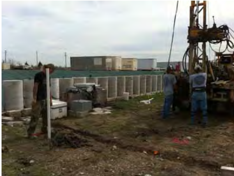
Figure 4.25: Piezometer being installed in borehole A.
