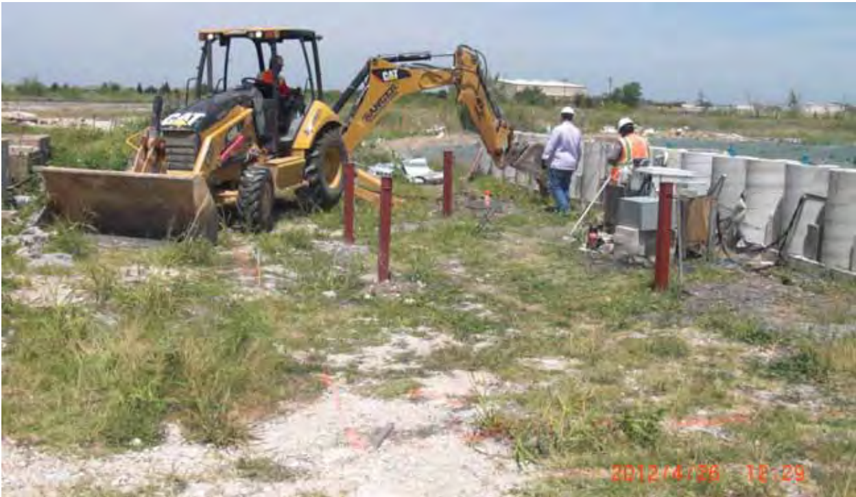
Figure 4.29: Excavation of trench for inundation berm.
