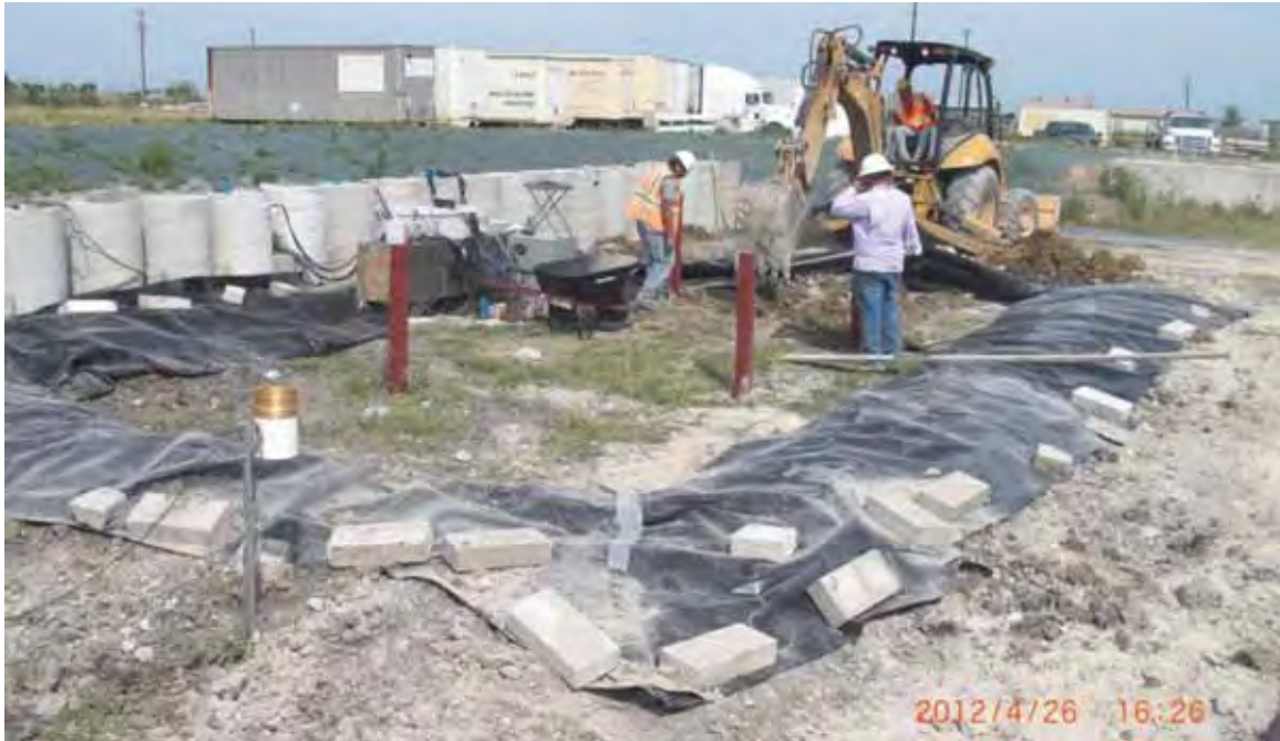
Figure 4.32: Compacting soil with backhoe bucket.
