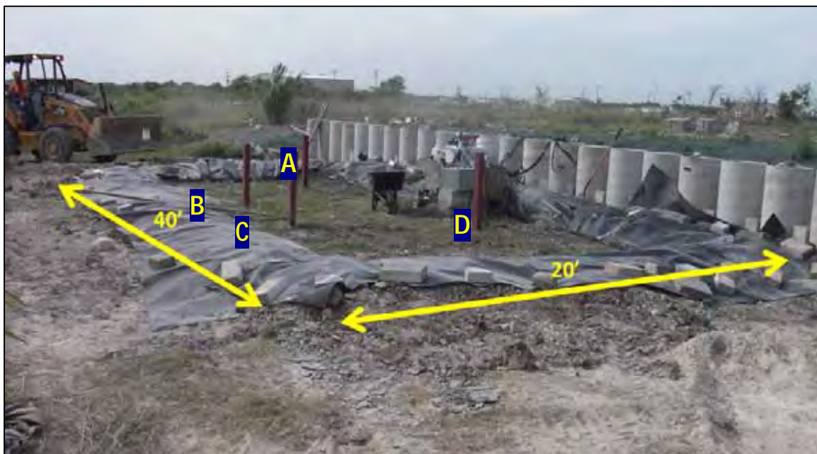
Figure 5.25: Inundation berm and stand pipe piezometers (April 26, 2012).
