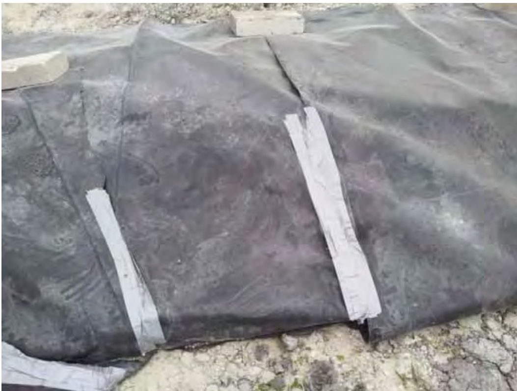
Figure 4.33: Detail of geomembrane seam.
