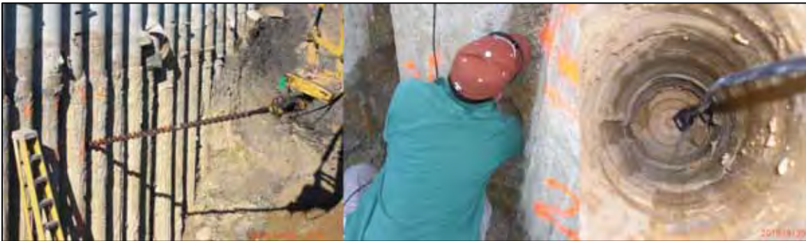
Figure 4.17: Installation of TDR moisture probes behind wall facing.
