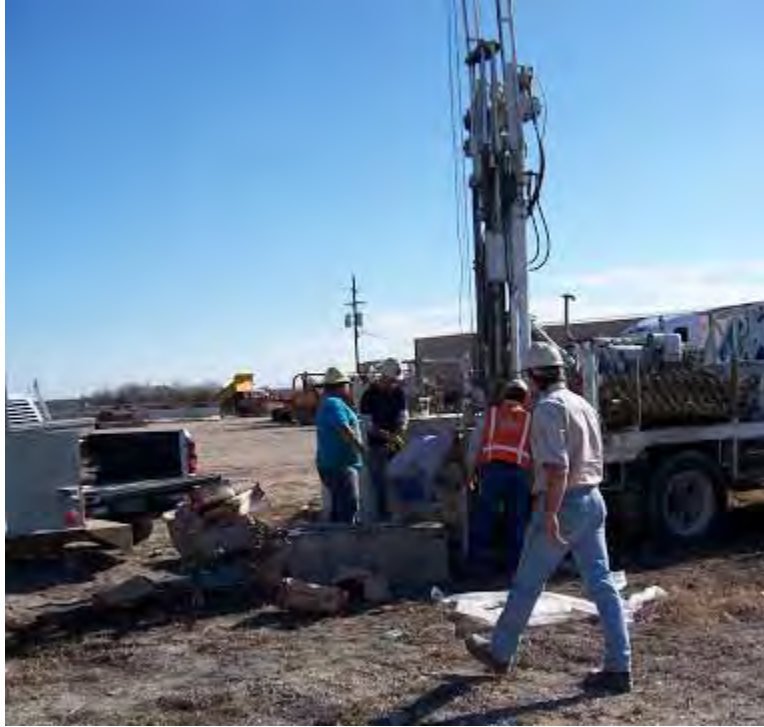
Figure 4.23: The piezometer installed in borehole B-3 being lowered into position.
