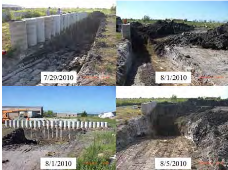
Figure 5.5: Photos of initial excavation progress (7/29/2010–8/5/2010).
