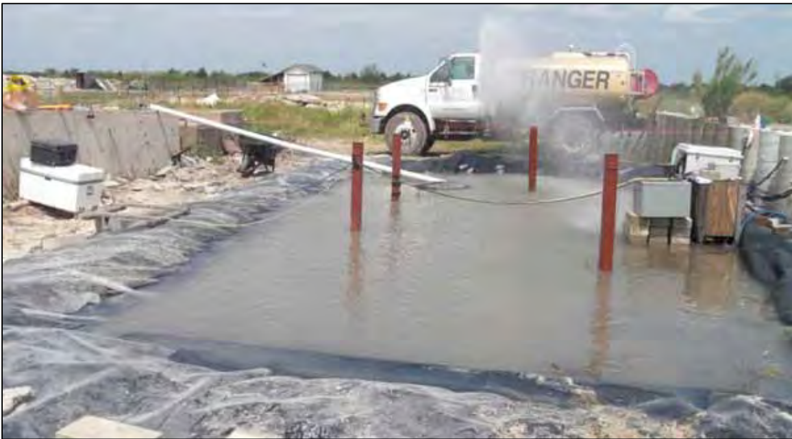
Figure 5.36: The inundation zone is filled on May 3, 2012.
