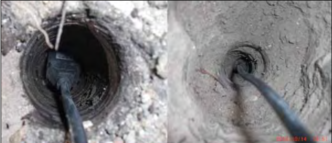
Figure 4.18: Installation of TDR moisture probes through ground surface.
