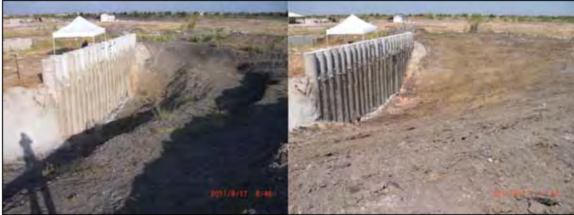
Figure 4.20: Excavation slopes are reshaped on August 17, 2011.
