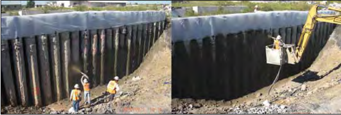
Figure 4.16: Installation of shotcrete facing on October 1, 2010.
