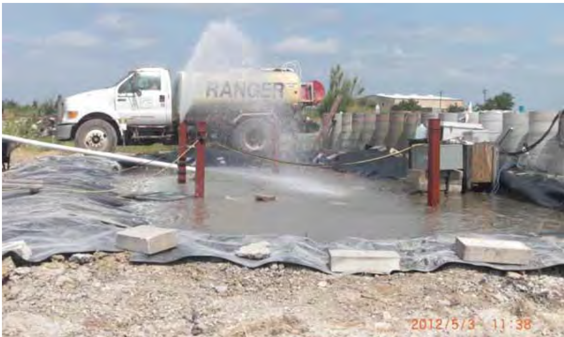
Figure 4.35: Filling the inundation zone.
