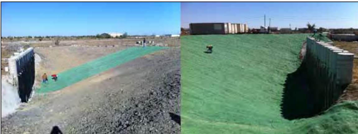
Figure 4.21: Erosion control material is installed on October 18, 2011.
