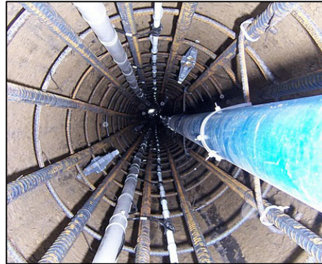
Figure 7: Instrumented Cage During Installation
