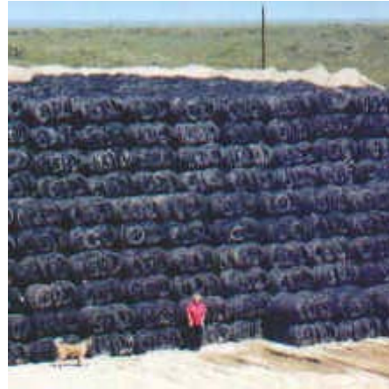
Figure 8.1: Stockpile of Tire Bales Ready to be Used in Construction
