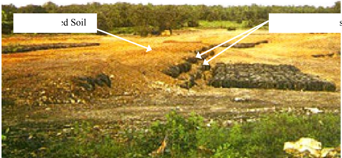
Figure 2.19: Tire Bales Used as a Fill Material in the Outer Shell of an Earthen Dam ( http://www.eagle-equipment.com/enviroblock.html )
