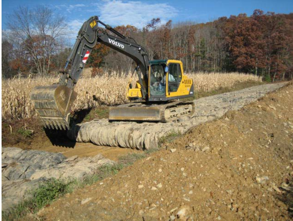
Figure 2.15: Use of Tire Bales as Roadway Subgrade in Pennsylvania ( www.dep.state.pa.us/dep/deputate/pollprev/starrTirePile/Images/IMG_0193 )
