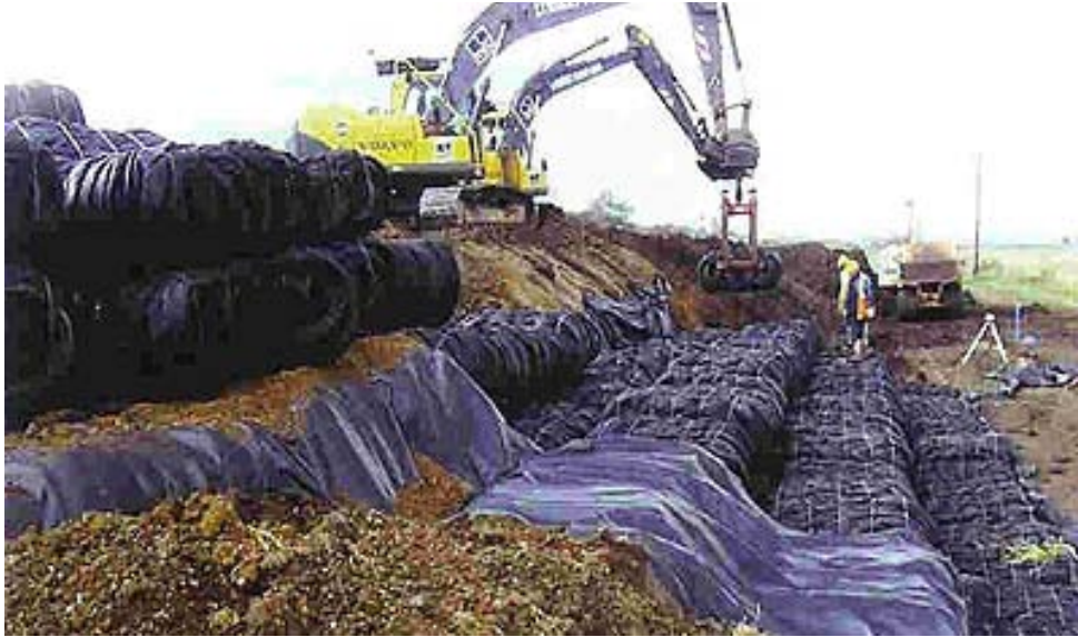
Figure 2.22: Proposed Expansion to Flood Embankment ( www.angloenvironmental.com/tyre_blocks_anglo.php )
