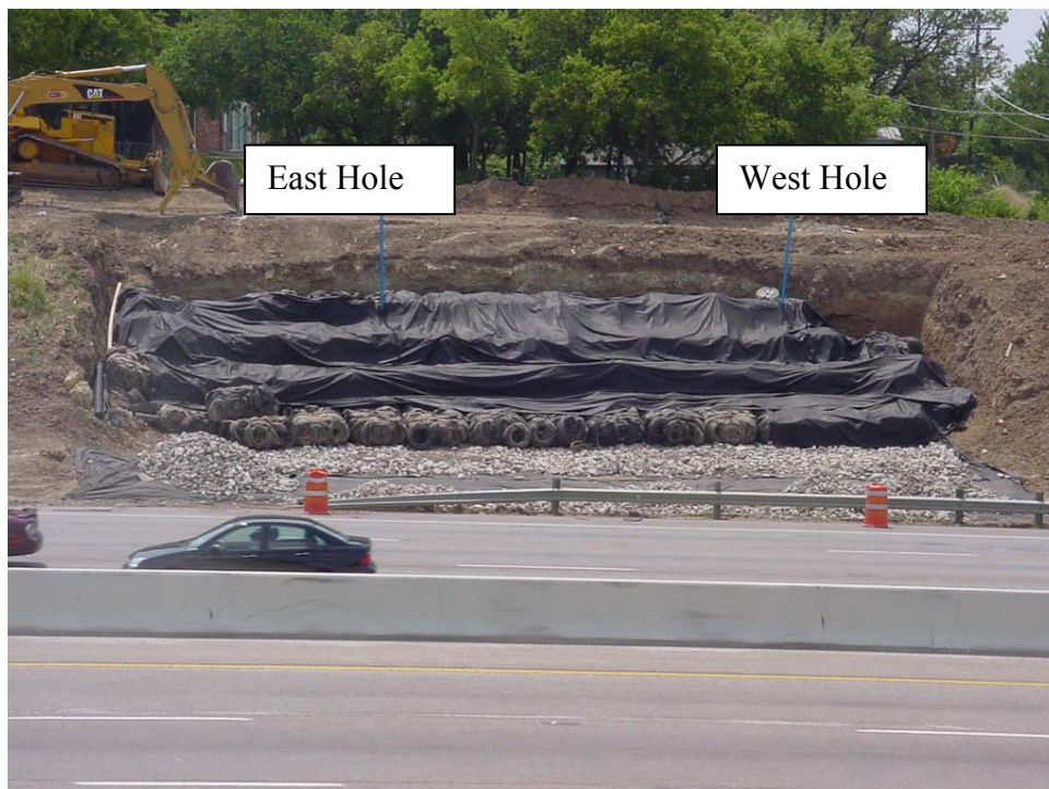
Figure 9.4: Tire Bale Components, Including the Two Inclinometers, for Phase Two Remediation
