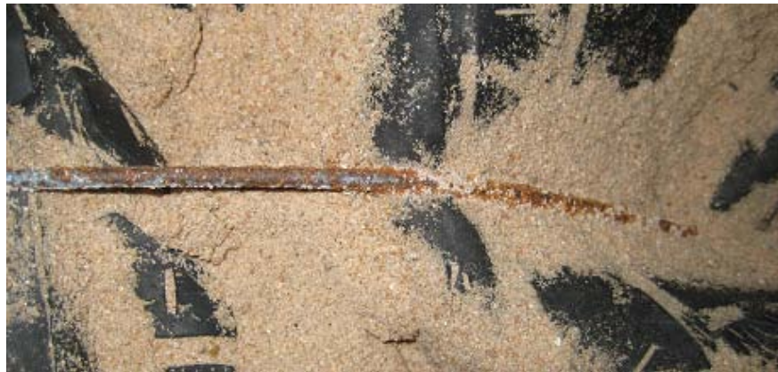
Figure 5.9: Corrosion of the Steel Baling Wires After Placement in a Wet Sand Fill
