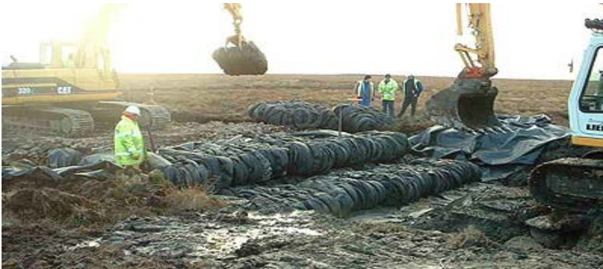
Figure 2.14: Lightweight Tire Bale Road Construction ( www.angloenvironmental.com/tyre_blocks_anglo.php )
