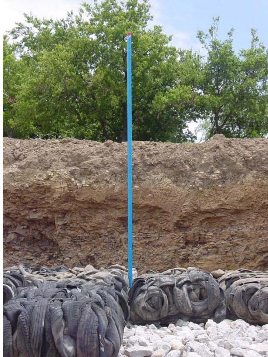
Figure 9.3: Inclinometer Tube Installed at the Base of the Phase Two Tire Bale Slope
