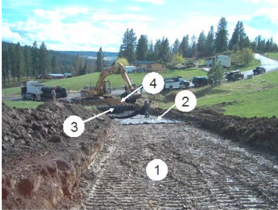
Figure 2.16: Photograph of a Roadway with a Single Layer Tire Bale Subgrade ( www.lstire.com/images/bale_job_during_resized.jpg )
