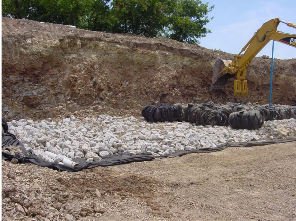
Figure 9.1: Gravel Drainage Layer and Pipe Drain for the Phase Two Remediation
