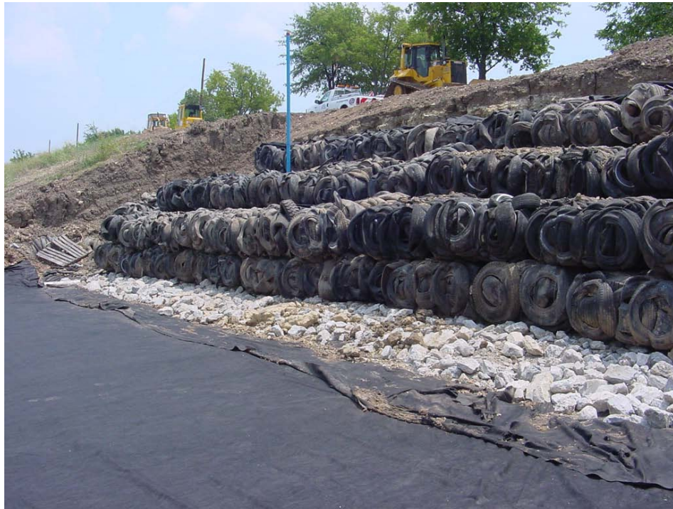
Figure 9.2: Tire Bale Mass for Phase Two Remediation (No Soil Infill between Layers)
