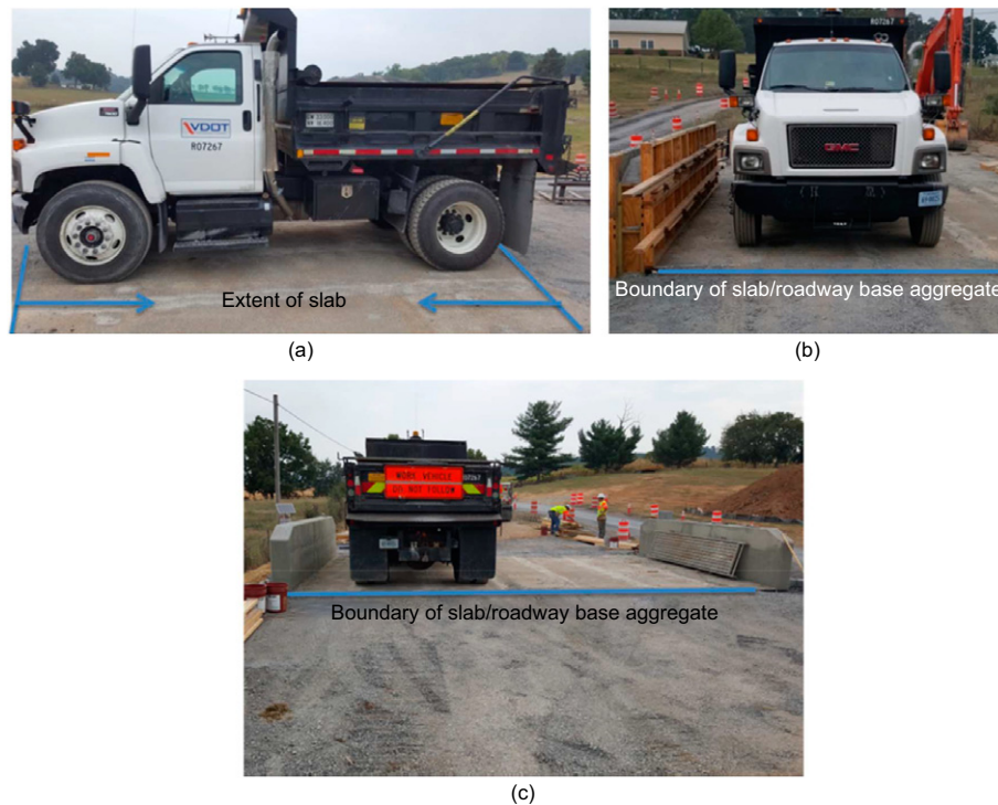
Figure 11. Truck loading on the superstructure after construction: (a) side view; (b) front view; and (c) rear view. Note: Truck was parked on each lane
