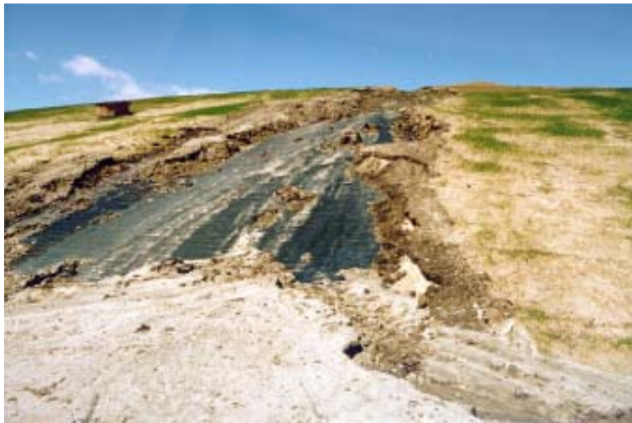
Figure 6-5. Poor cover design, resulting in both surface-water erosion failure (left) and sloughing of cover system due to excess buildup of pore water in cover drainage layer (below).
