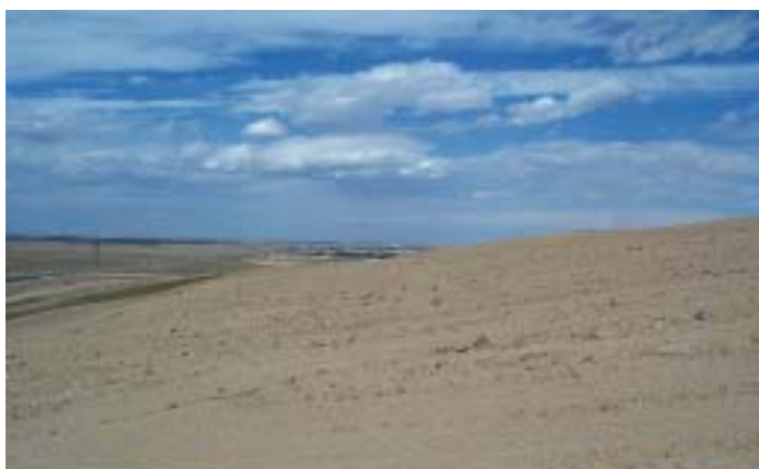
Figure 5-3. Topsoil layer at Denver Arapahoe Disposal Site before fine-grading and seeding.
