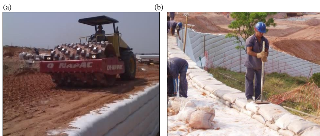
Figure 2. (a) Compaction and (b) soil bag facing construction.
