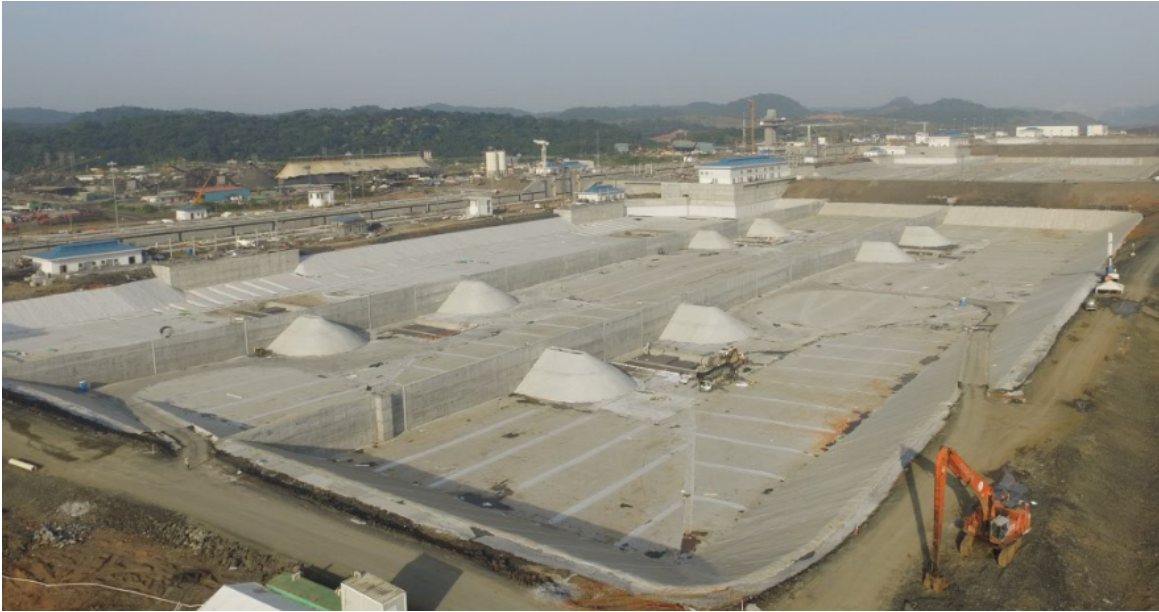
Figure 4: General View of Lower Chamber in the Pacific Site
