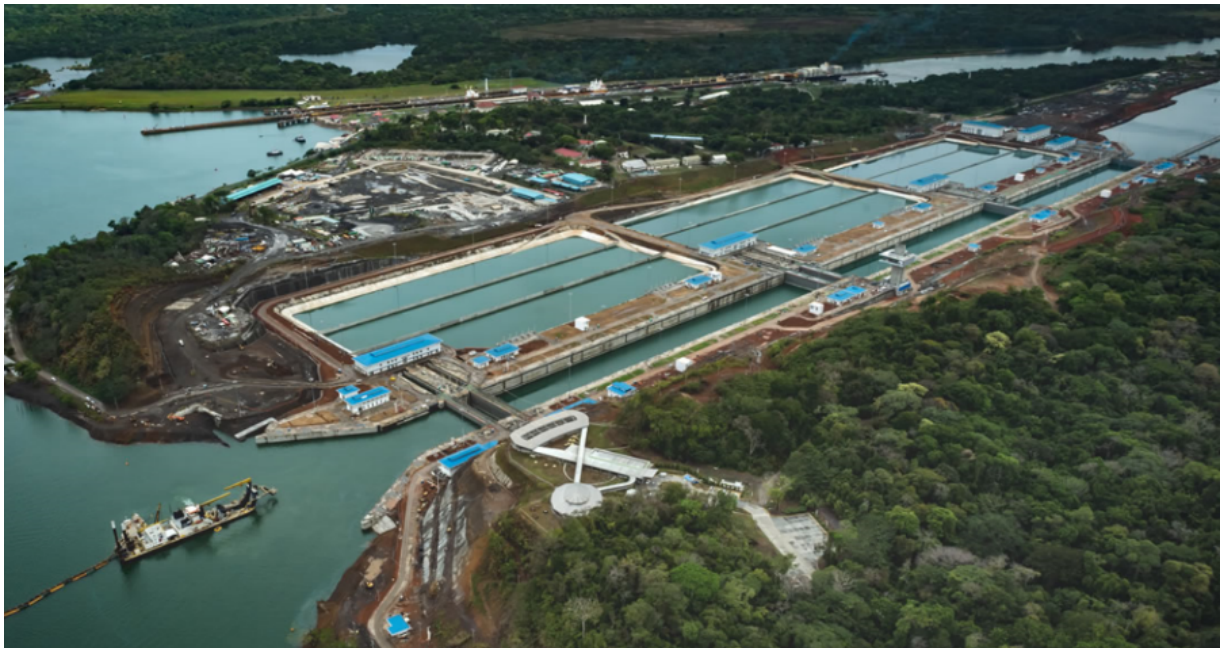
Figure 3: General View of the Atlantic locks
