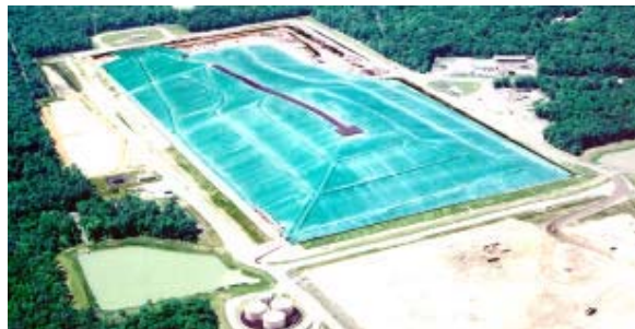
Figure 18. Exposed geomembrane cover over Cells 1 and 2 of the DSWA's southern facility.
