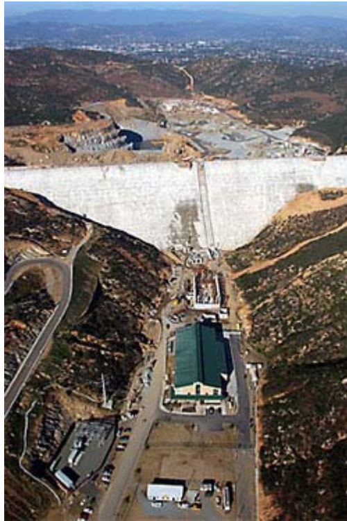
Figure 3. Olivenhain dam, an RCC Dam in California.
