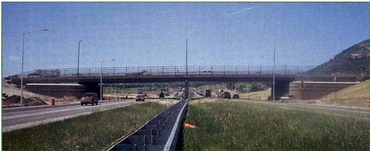
Figure 11. View of the Founders/Meadows GRS bridge abutments near Denver, Colorado.
