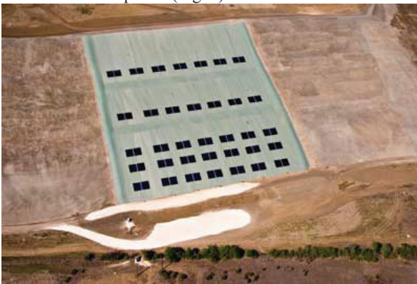
Fig. 2. Aerial view of the exposed geomembrane with arrays of solar panels at the Tessman Road Landfill (Roberts 2010)
