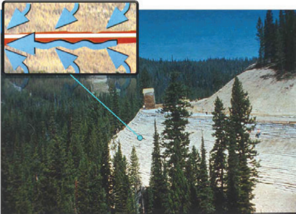
Fig. 10. Geosynthetic-reinforced slope in the Idaho National Forest, illustrating the use of reinforcement with in-plane drainage capabilities (Zornberg et al. 1997)
