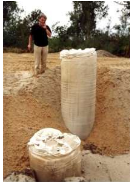
Fig. 7. View of exposed Geotextile Encased Column (Alexiew et al. 2011)
