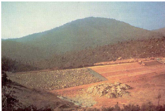
Fig. 1. Construction of the downstream drain of Valcros Dam (Giroud 1992)
