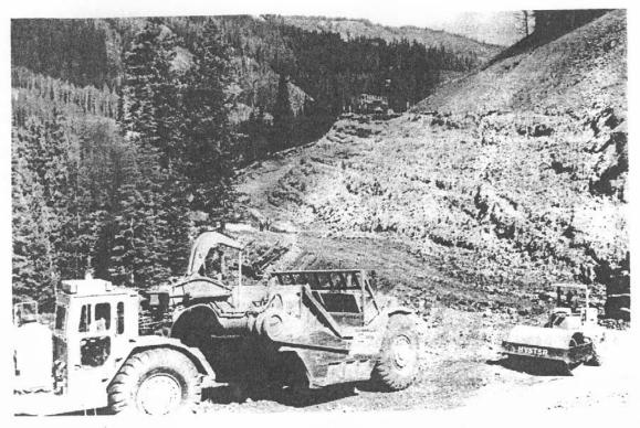
Figure 3. Rock shear key under construction
