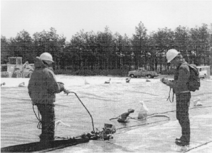
FIGURE 27.9 Monitoring seaming of a geomembrane liner.
