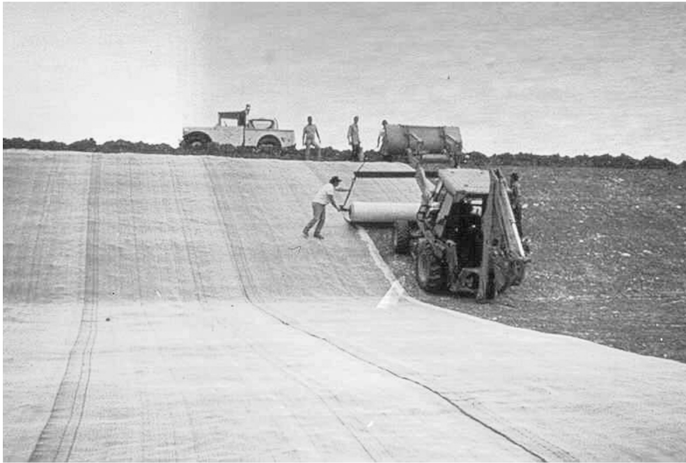
FIGURE 37.11 Installation of a GCL during construction of a landfill base liner.
