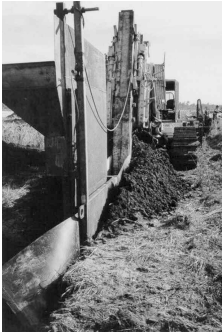
FIGURE 37.18 One pass trencher for installation of an HDPE vertical barrier system. (Photo courtesy of Groundwater Control, Inc.)
