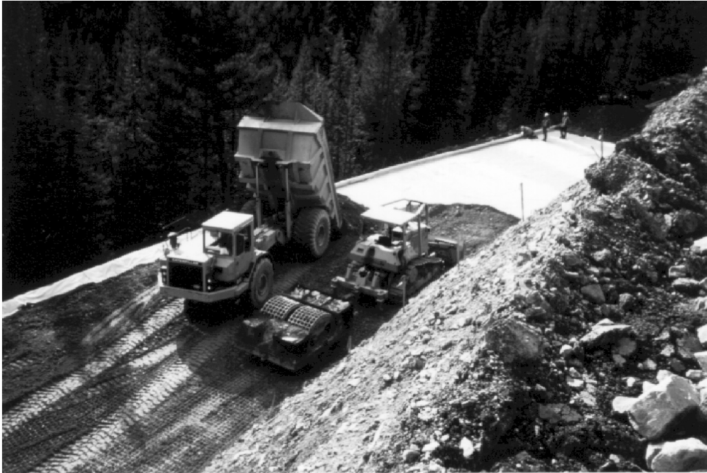
FIGURE 37.6 Placement of a high-strength nonwoven geotextile to perform a dual function of reinforcement and in-plane drainage in a reinforced slope.
