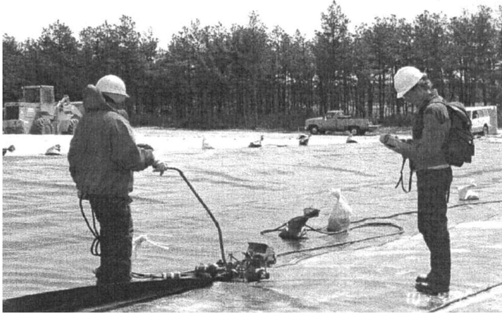
FIGURE 37.9 Monitoring seaming of a geomembrane liner.
