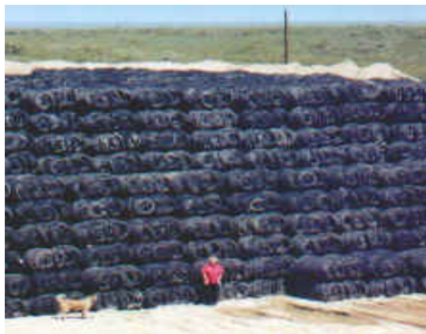
Figure 5.3. Stacked tire bales, e.g., to form the impact face of a rockfall barrier (Encore Systems, 2004)
