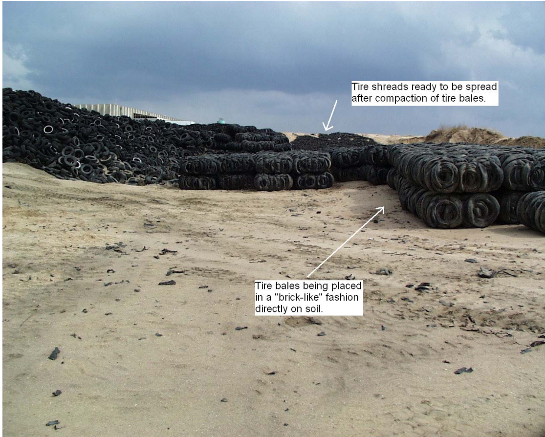
Figure B5. Roadway construction using tire bales.
