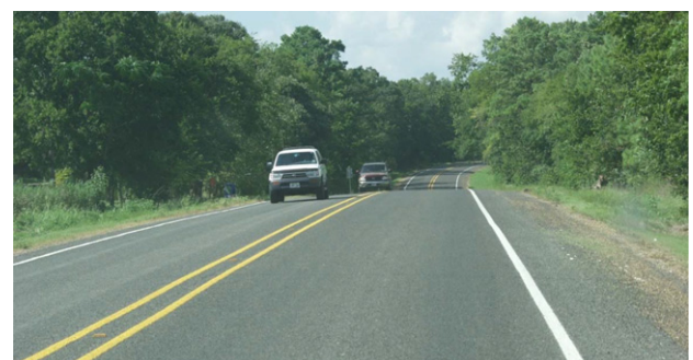
Figure 10. View of road conditions in 2004 at the FM1774 test section stabilized using GS1 in Case Study B
