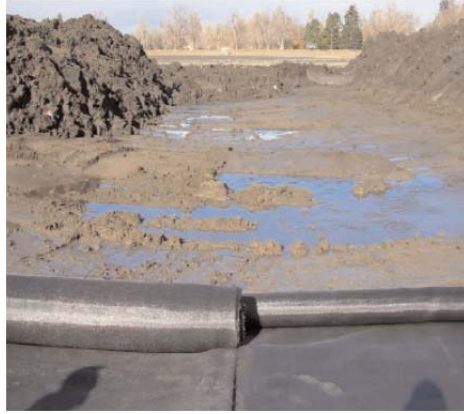
Figure A8: Placement of woven geotextile for subgrade restraint (Mirafi 2008)
