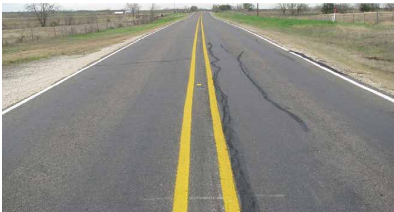
Figure 5. Road conditions showing control section (right) and geosynthetic-stabilized base section (left).
