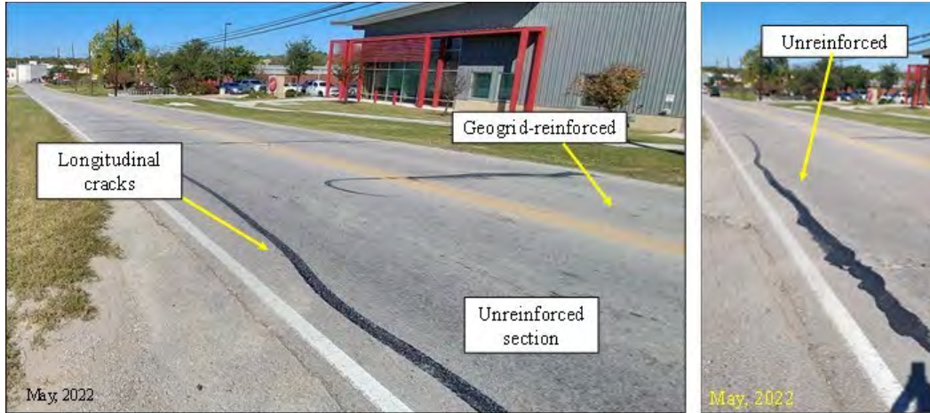
Figure 6. Road conditions during 2022 survey.
