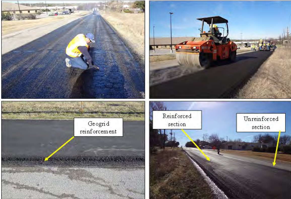
Figure 5. Final paving work at the geosynthetic-reinforced section.
