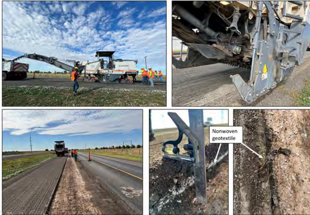
Fig. 2 - Milling operations to collect RAP and GRAP samples at US70/84 (July 2022).
