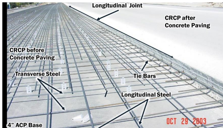
Figure 2.10: Construction details of CRCP in Texas (TxDOT, 2019).
