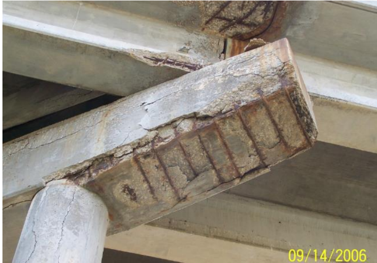
Figure 1.3: Leaking issues associated with expansion joints (Hyzak, 2021).
