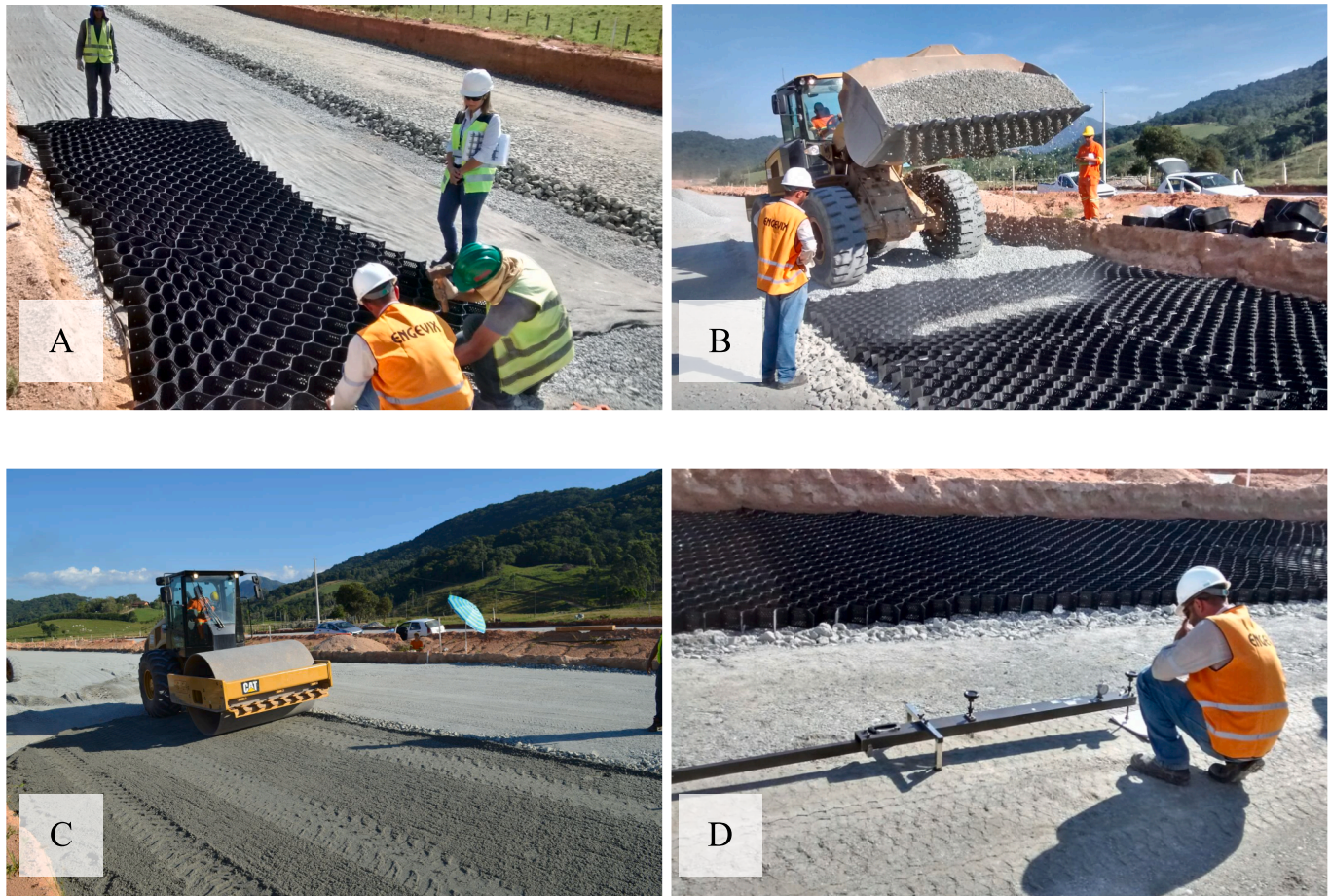
Fig. 3. Installation steps of geocell-reinforced zone 3: A) Geocell installation; B) Geocell filling; C) Layer compaction; and D) Deflection test (BBT).
