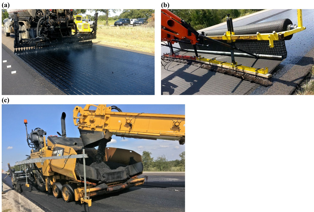
Fig. 3 SH21 rehabilitation: a Application of binder tack coat; b Installation of polymeric geosynthetic reinforcement; c Construction of asphalt overlay
