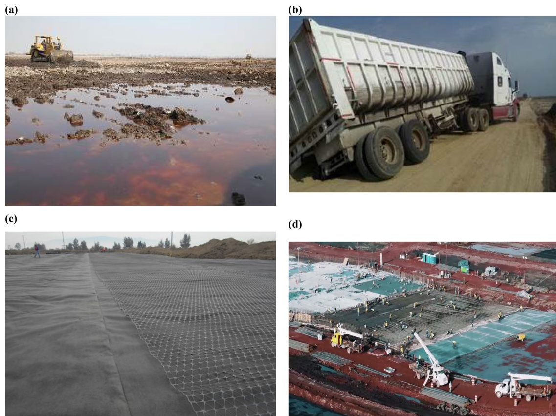
Fig. 19 Case study involving stabilization of soft subgrade: a View of the saturated clay at the New International Airport of Mexico City before construction; b Evidence of significant problems with low
