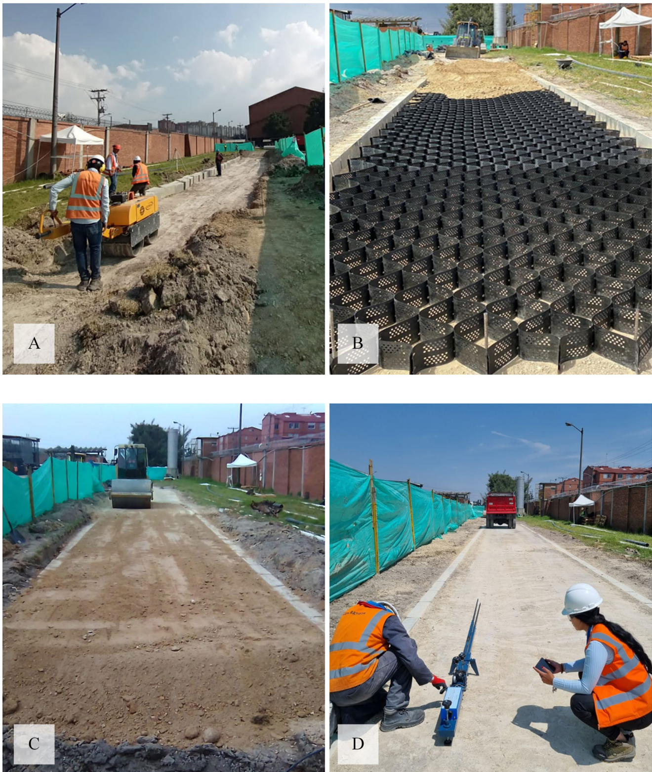
Fig. 2 Test Sections construction: A) base layer preparation; B) filling of geocell-reinforced layer; C) compaction operations; and D) deflection test (BBT) being conducted on one of the constructed layers
