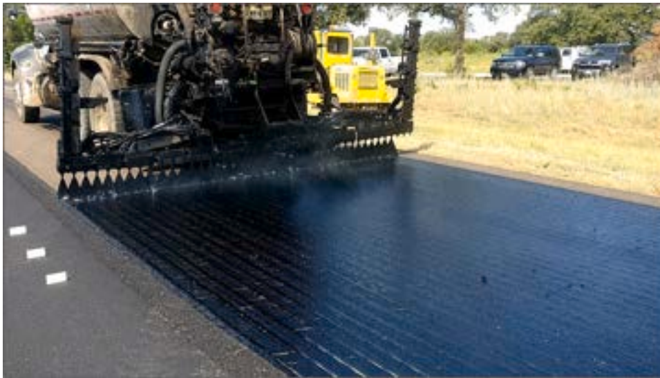
Fig. 8. Polymer asphalt cement (AC-15P) tack application in experimental test section.
