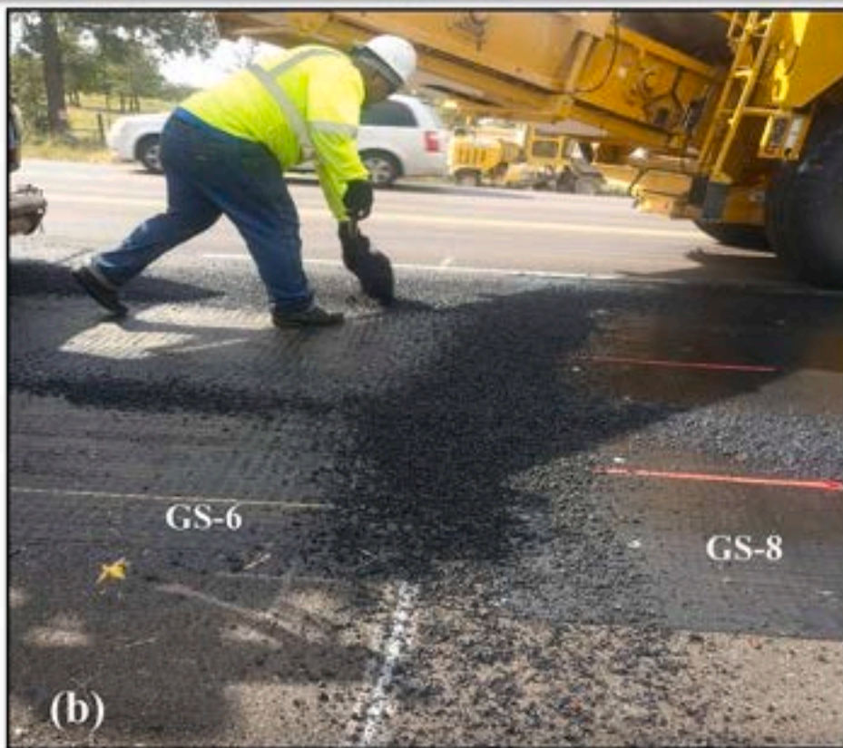
Fig. 20. Asphalt sanding: (a) uphill paver wheel path; and (b) geosynthetic overlap.
