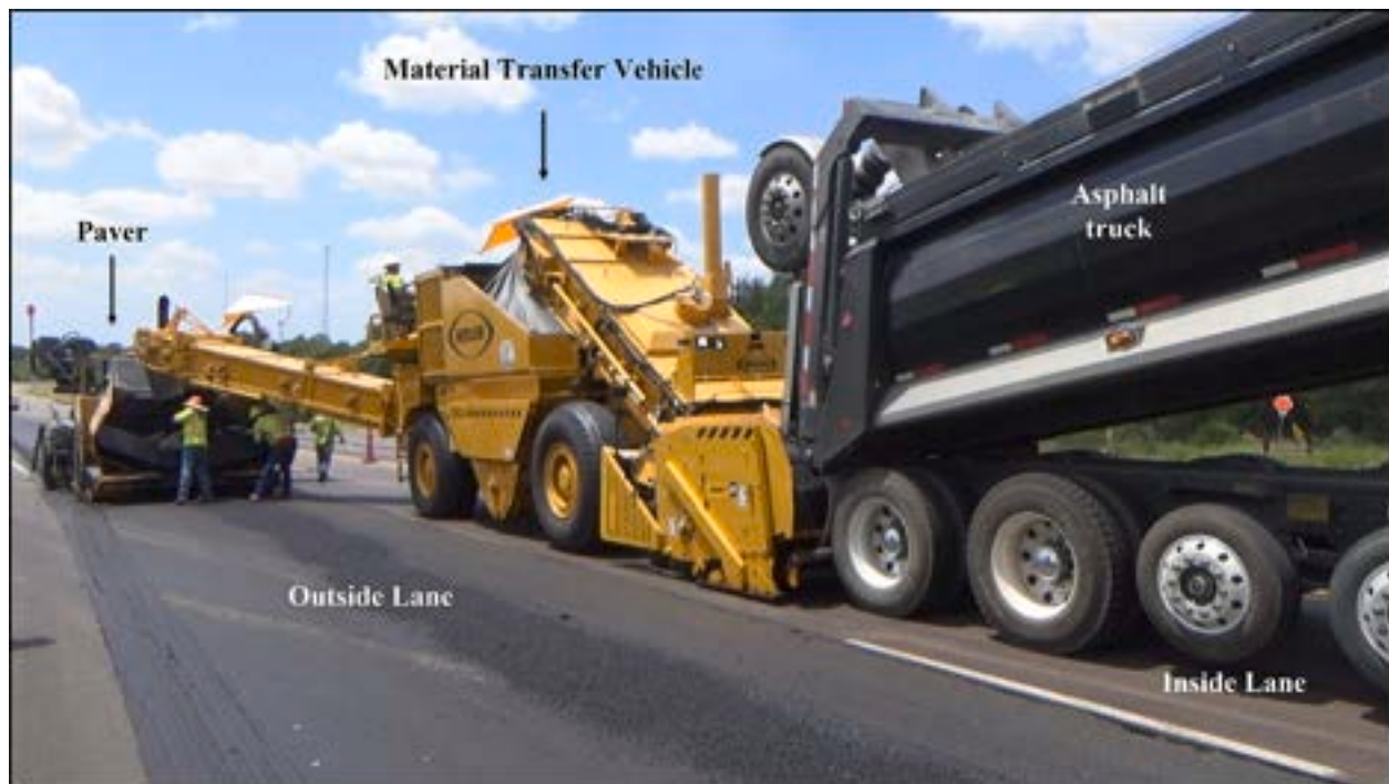
Fig. 17. Revised overlay construction process.
