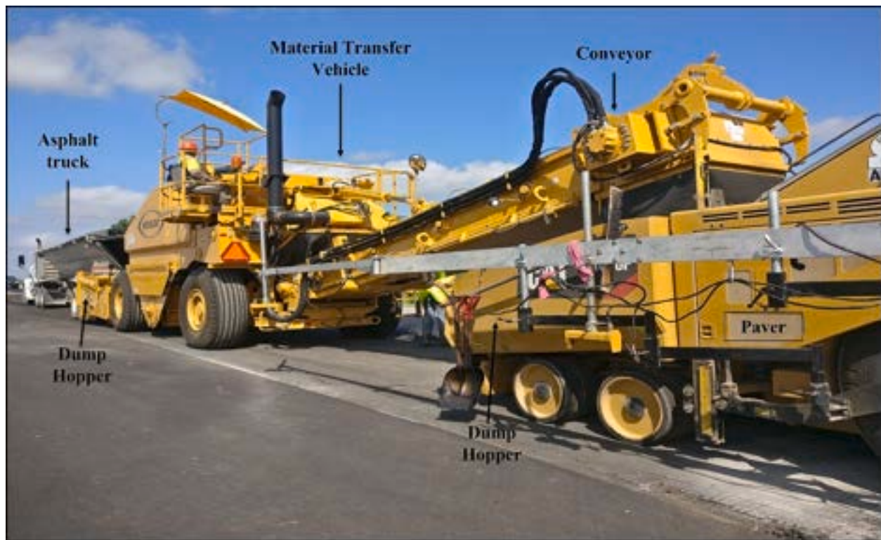
Fig. 14. Asphalt overlay construction equipment used in SH21 rehabilitation project.
