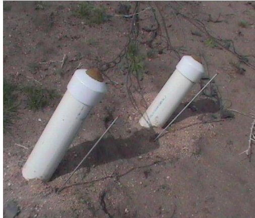
Figure 25: Placement of the PVC Pipes in the Layered Section Following Construction
