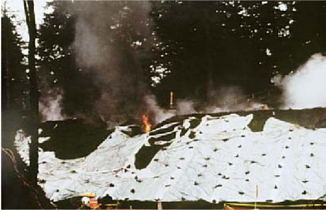
Figure 3: SR 100 Tire Shred Embankment during Removal
