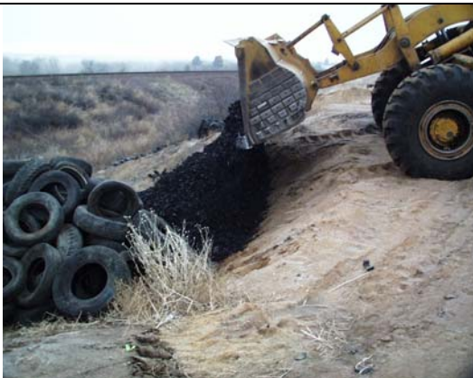
Photo A-15: Construction of Tire Shred-Only Stockpile
