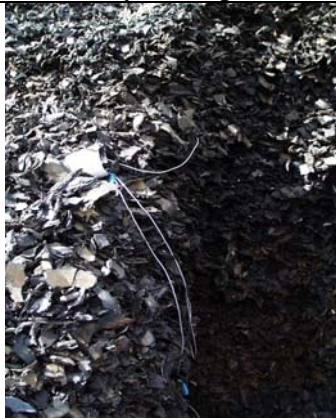
Photo A-27: Detail of Instrument Wiring in the Large Tire Shred-Only Stockpile
