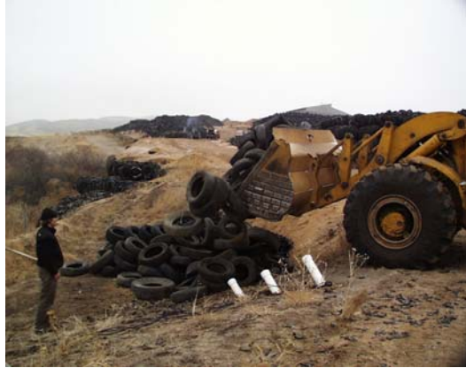
Photo A-14: Construction of Whole Tire Stockpile
