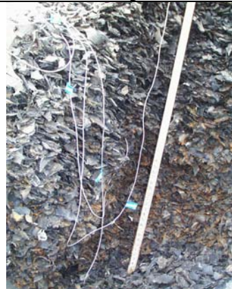
Photo A-28: Installation of Thermistor in the Large Tire Shred-Only Stockpile
