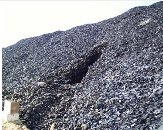
Photo A-22: View of Large Tire Shred-Only Stockpile and Ditch Constructed for Instrumentation Installation
