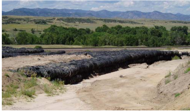
Figure 13: Front Range Tire Recycle, Inc. Tire Bale Embankment
