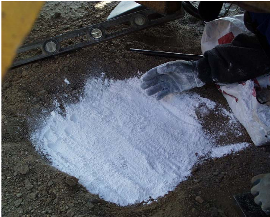
Figure 37: Plate-load test area after placement of plaster
