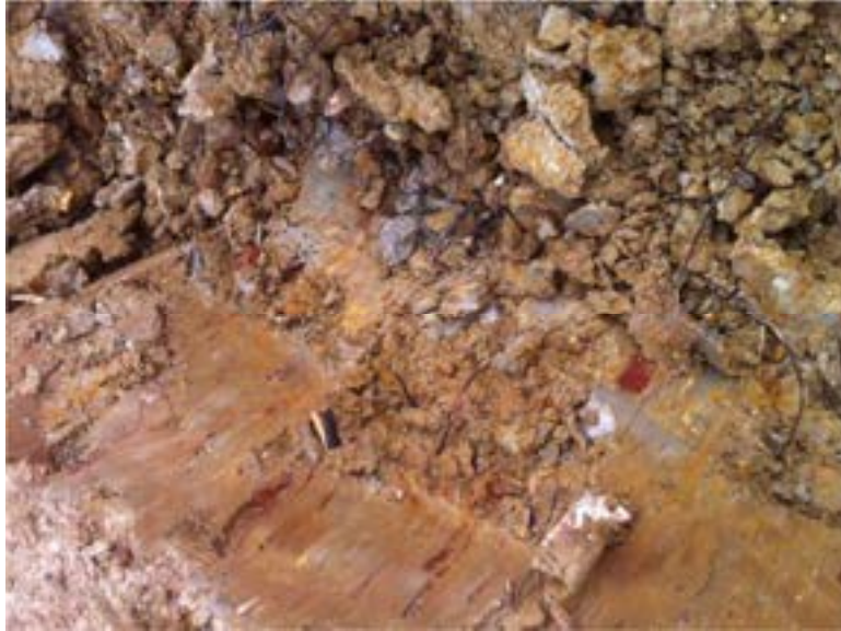
Figure 4.69: Cut in Cook Mountain Clay during Sensor Installation
