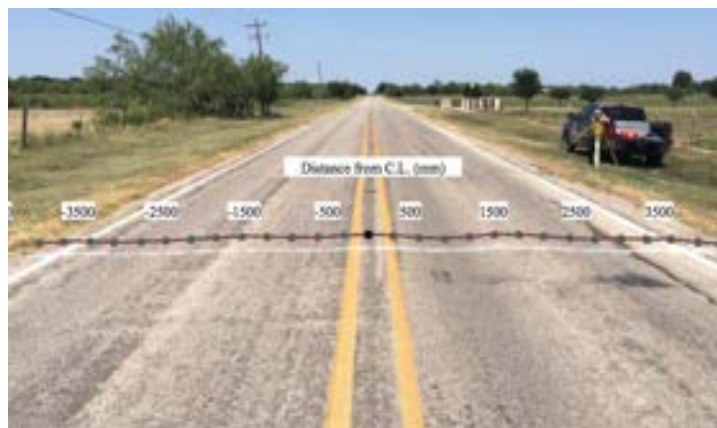
Figure 5.53: Total Station Marking
