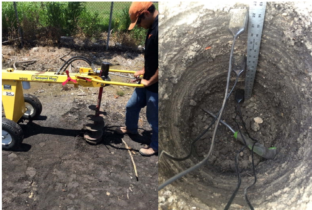
Figure 5.51: Installation of Field Sensors at Inundation Project
