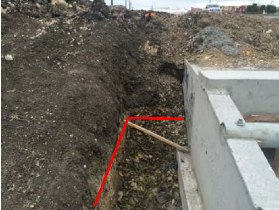
Figure 5.42: FM 685 Soil Deposits prior to Sensor Installation
