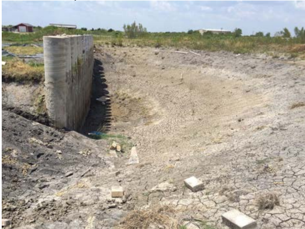
Figure 4.9: Manor Retaining Wall Site in August 2015
